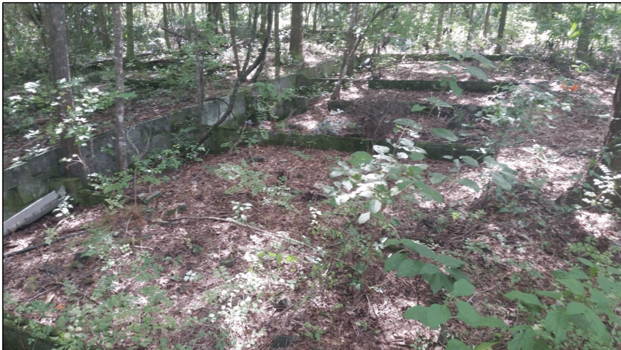
Figure 32. Old foundation located in the central portion of the study site.
