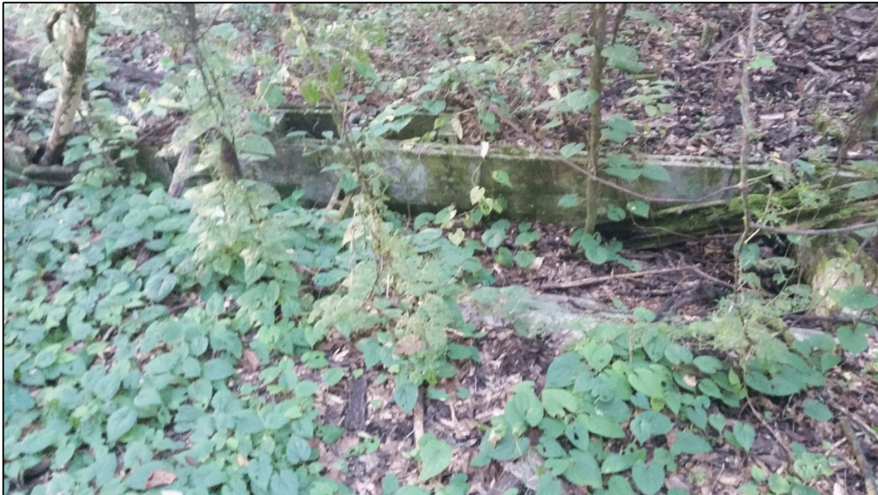
Figure 30. Old foundation located in the parcel 06949-000-000
