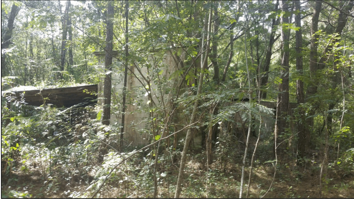
Figure 37. A dilapidated structure in the central areas of the study site.
