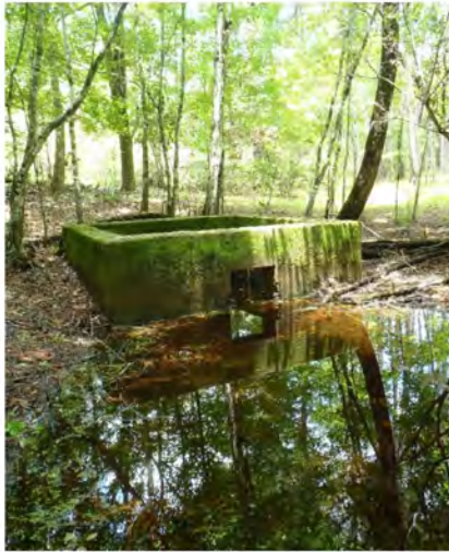
Photo 9. Exterior view of Blues Creek overflow structure (GPS 820).
