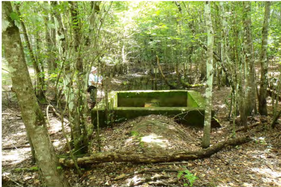
Photo 6. Blues Creek overflow structure located on west side of spillway (GPS 820).
