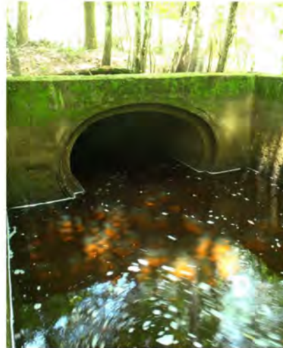
Photo 10. Interior view of Blues Creek overflow structure (GPS 820).
