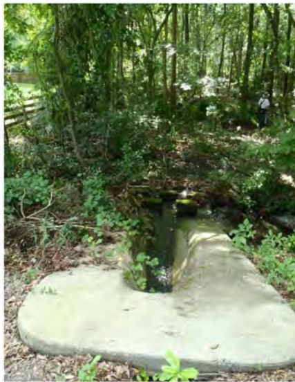
Photo 50. Major stormwater inflow structure (GPS 1394).
