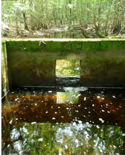
Photo 7. Interior view of Blues Creek overflow structure (GPS 820).
