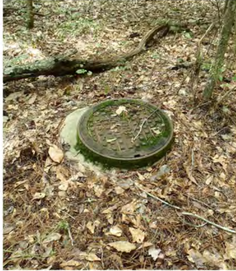
Photo 57. Stormwater manhole cover (GPS 1201).
