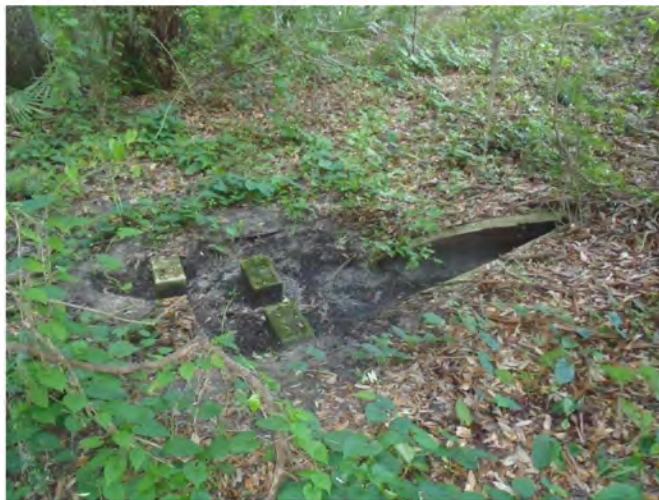
Photo 62. Stormwater inflow culvert (GPS 1276).
