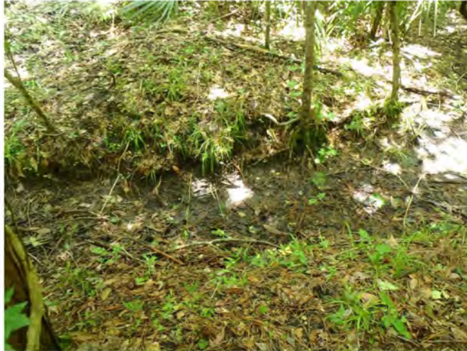
Photo 28. Breach in berm (GPS 955).
