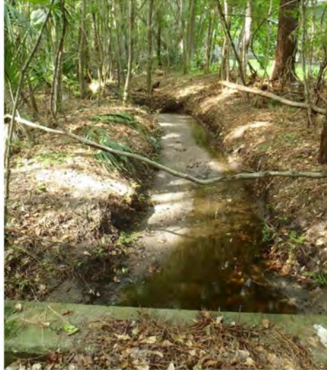
Photo 59. View downstream from culvert (GPS 1202).
