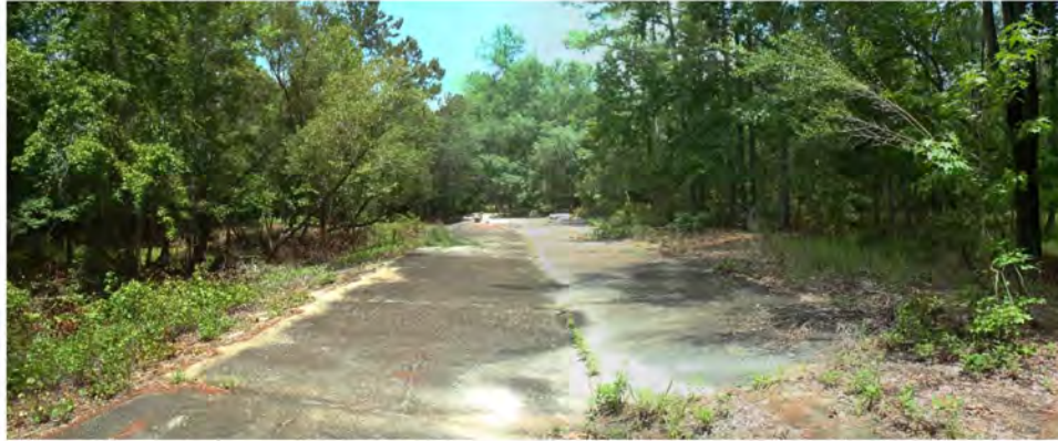
Photo 5. Blues Creek spillway structure (GPS 820).
