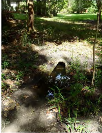
Photo 49. Stormwater draining into swamp (GPS 1393).
