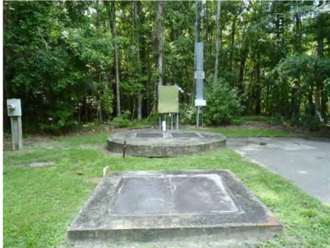
Photo 55. Lift station (GPS 1198).
