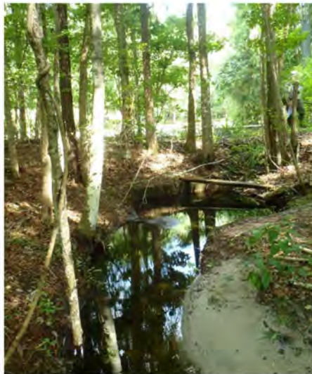
Photo 54. Culvert and headwall (GPS 1186).
