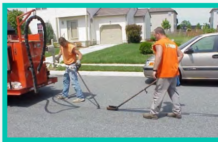
Crack Sealing
