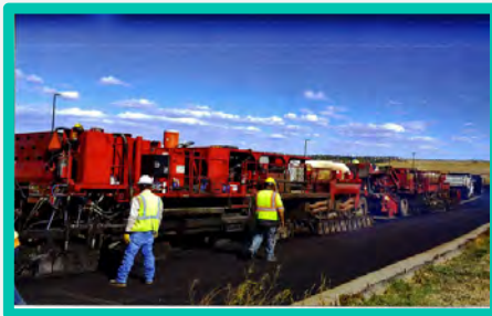
Hot In-Place Recycle
