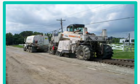
Full Depth Reclamation / Reconstruction
