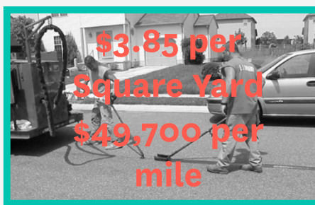
Crack Sealing
