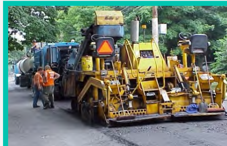
Cold In-Place Recycle
