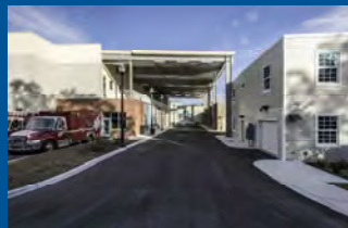
Kirkpatrick Center Institute of Public Safety Gainesville, FL
