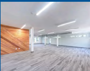
Catalyst Park Interior Renovations Gainesville, FL
