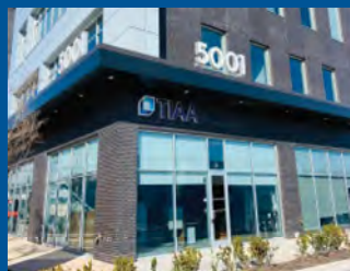
TIAA Bank, Buildout Gainesville, FL
