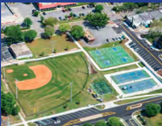
Alachua Roadway and Stormwater Improvements Alachua, FL
