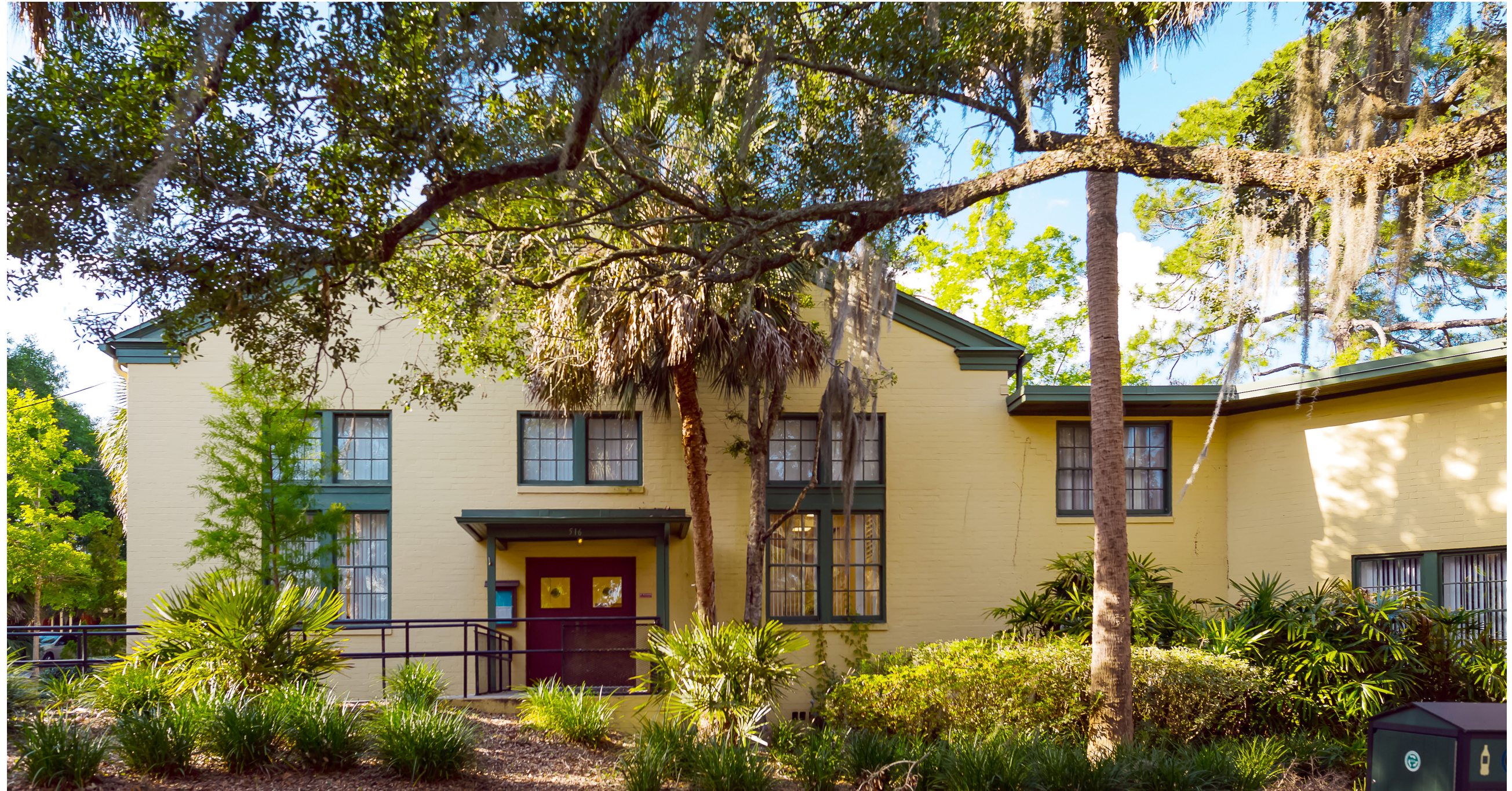
Thelma Boltin Center Existing South Entrance
