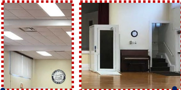
Existing building finishes & ADA access to stage
