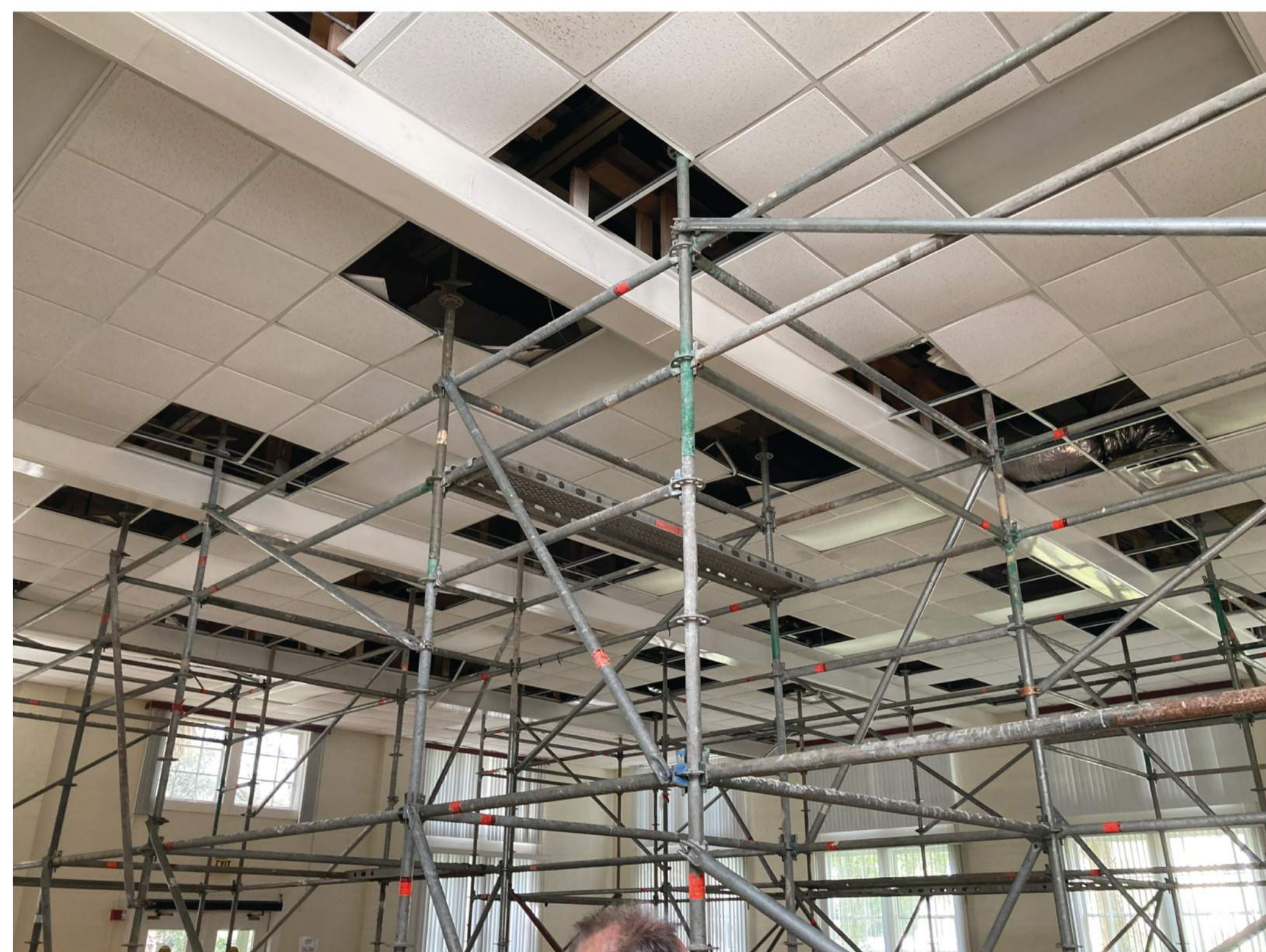
3 FIRST FLOOR AUDITORIUM CEILING
