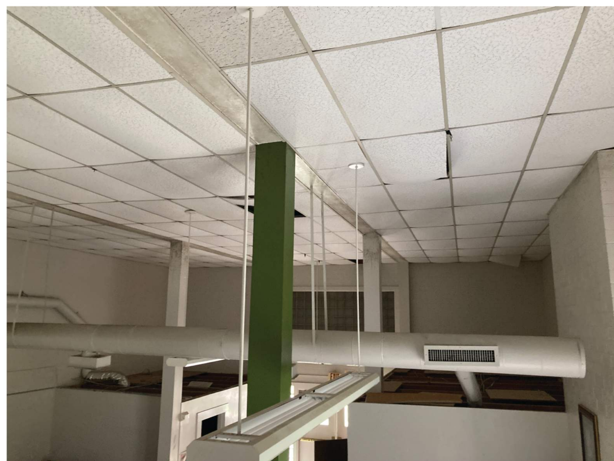
3 FIRST FLOOR GROUP ROOM CEILING
