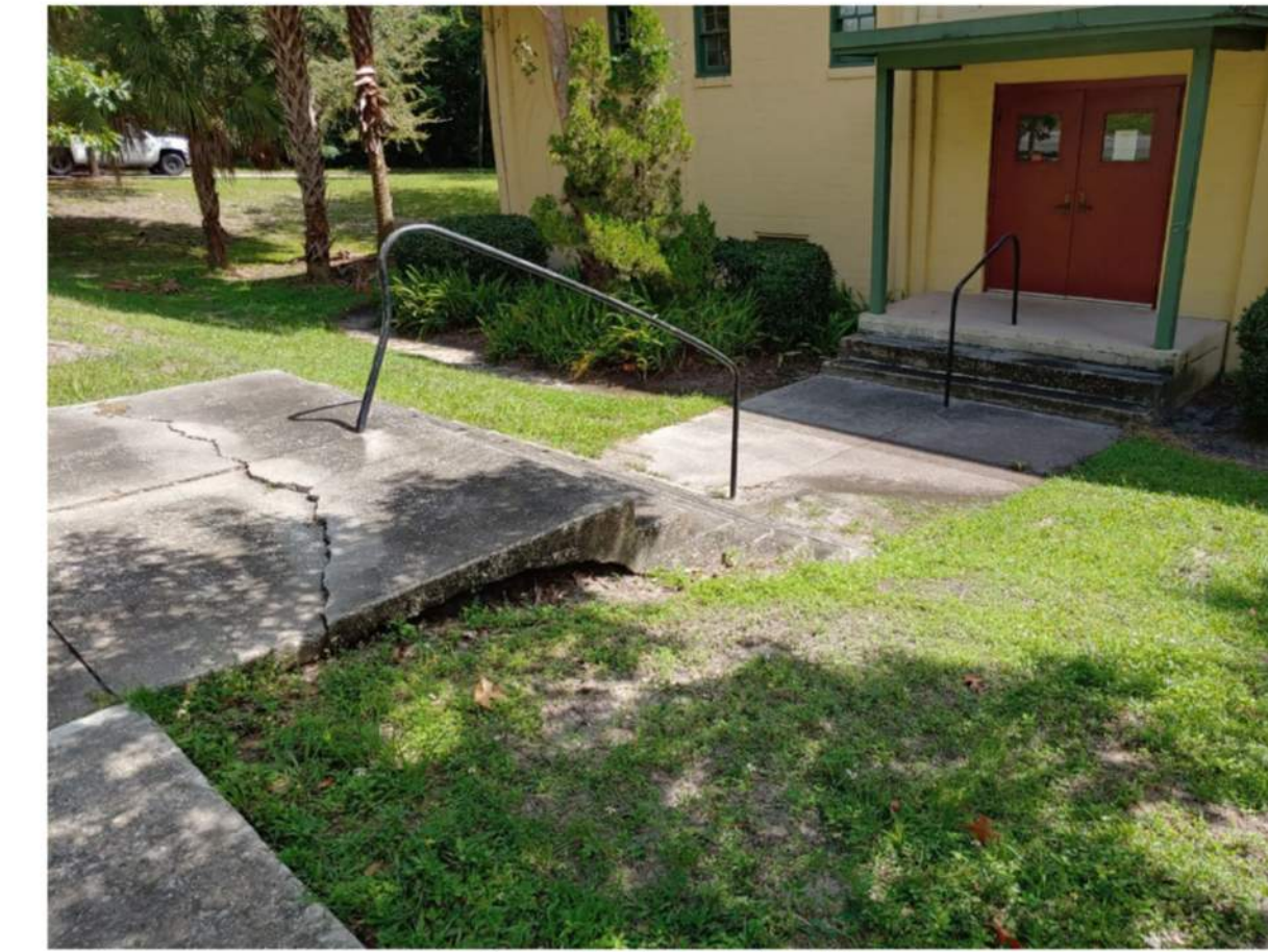
Figure 2. Stairway Undermining
