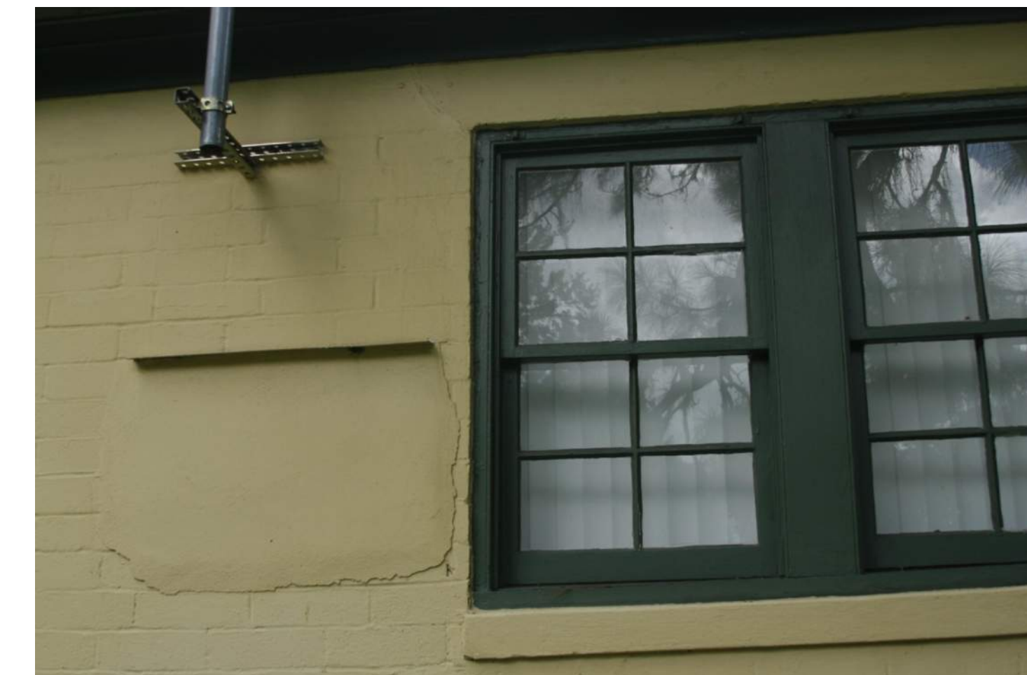
6 WALL PATCH AT EAST
