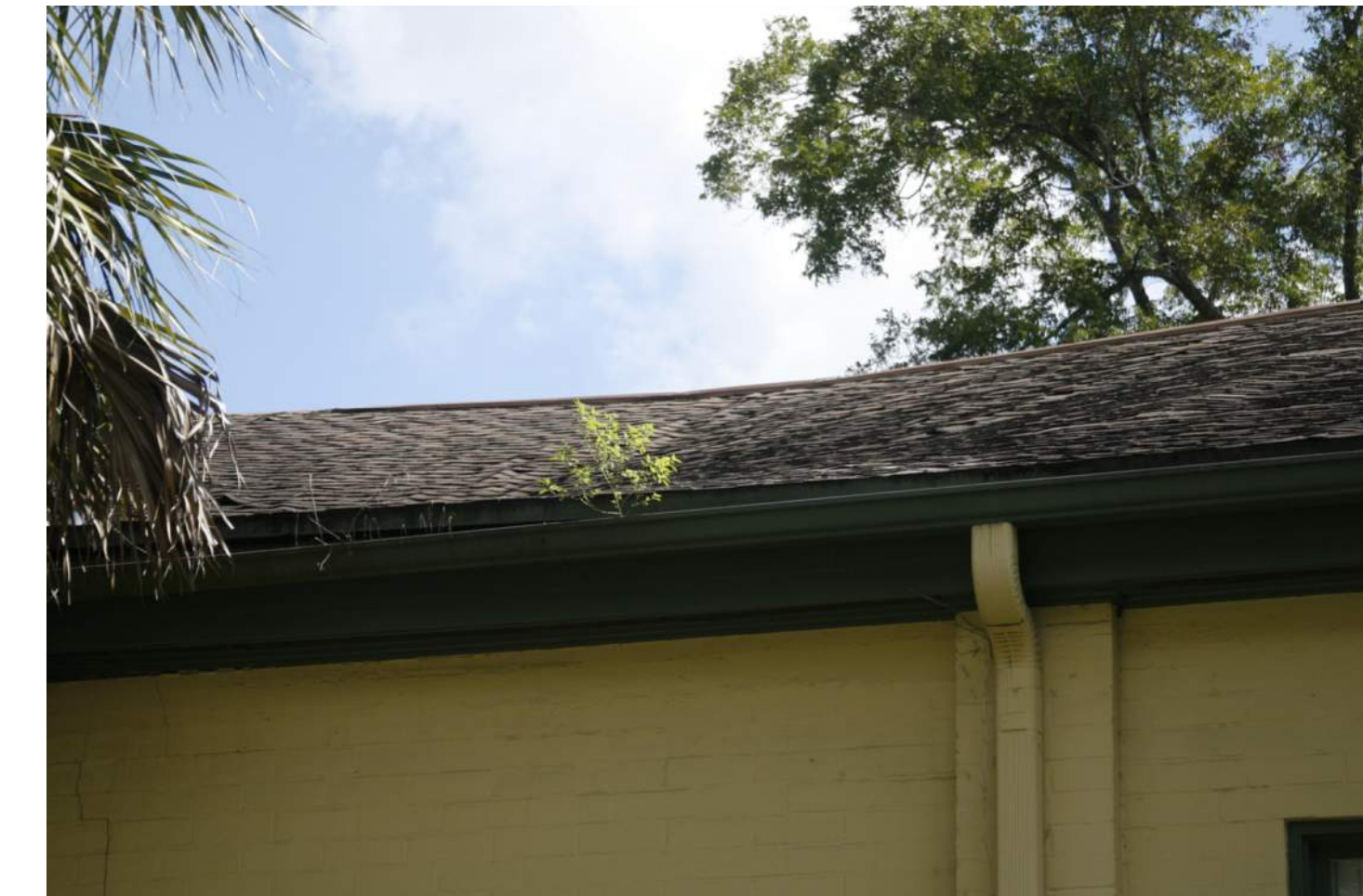
3 GUTTER AND ROOF CONDITIONS AT WEST
