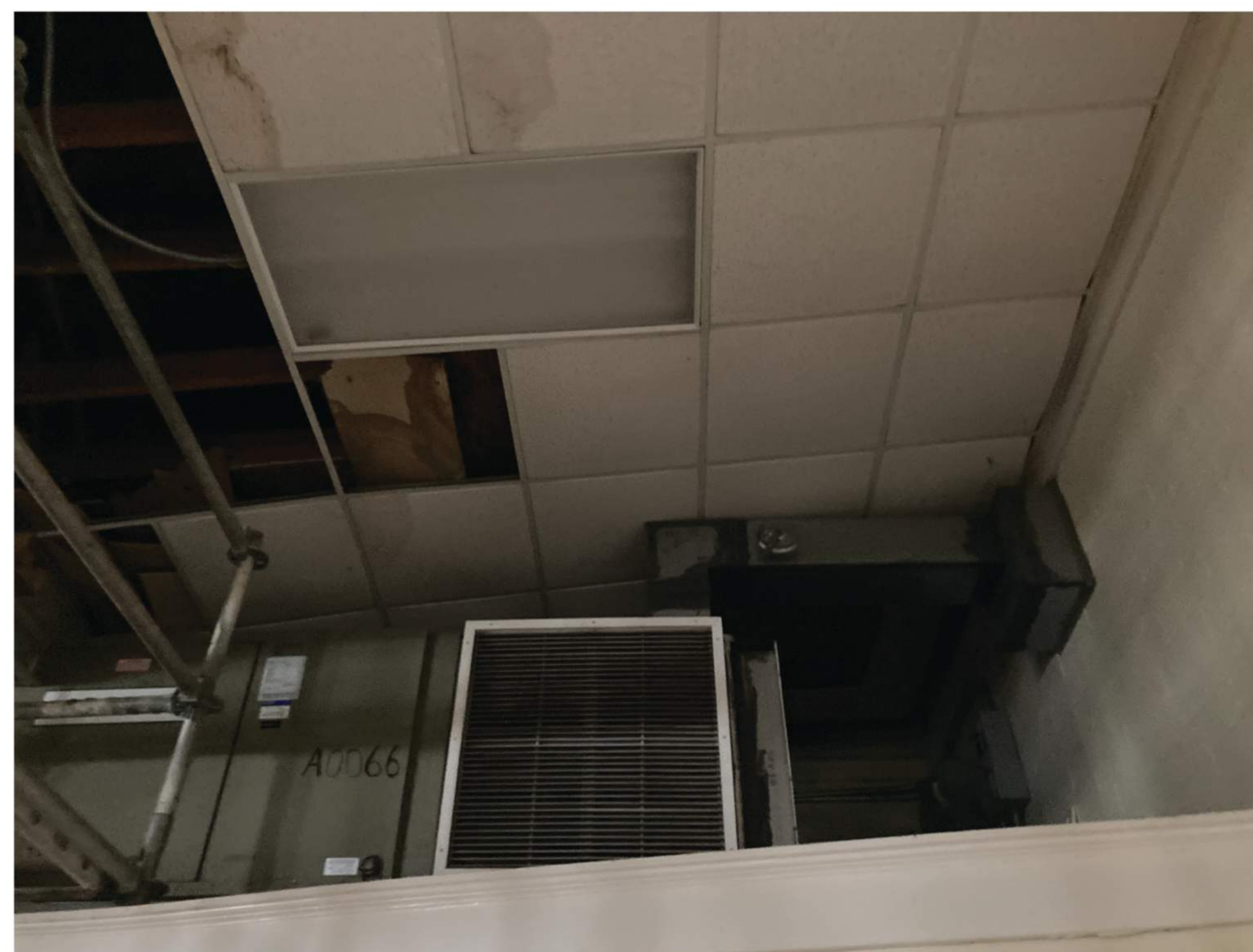
4 STAGE CEILING, FIRST FLOOR
