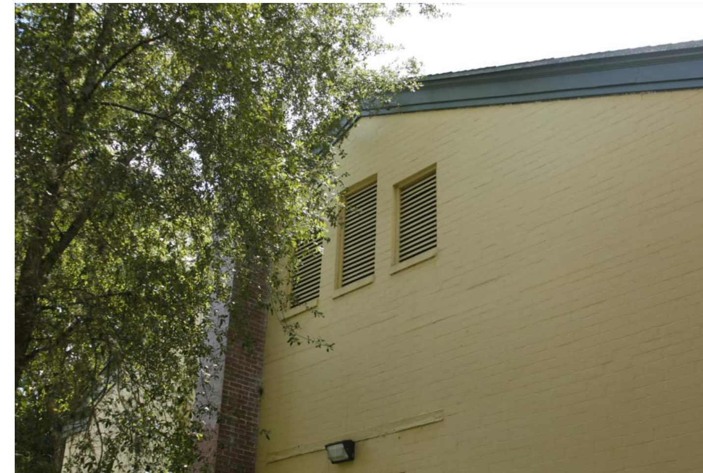
2 CHIMNEY AND ATTIC VENTS AT NORTH
