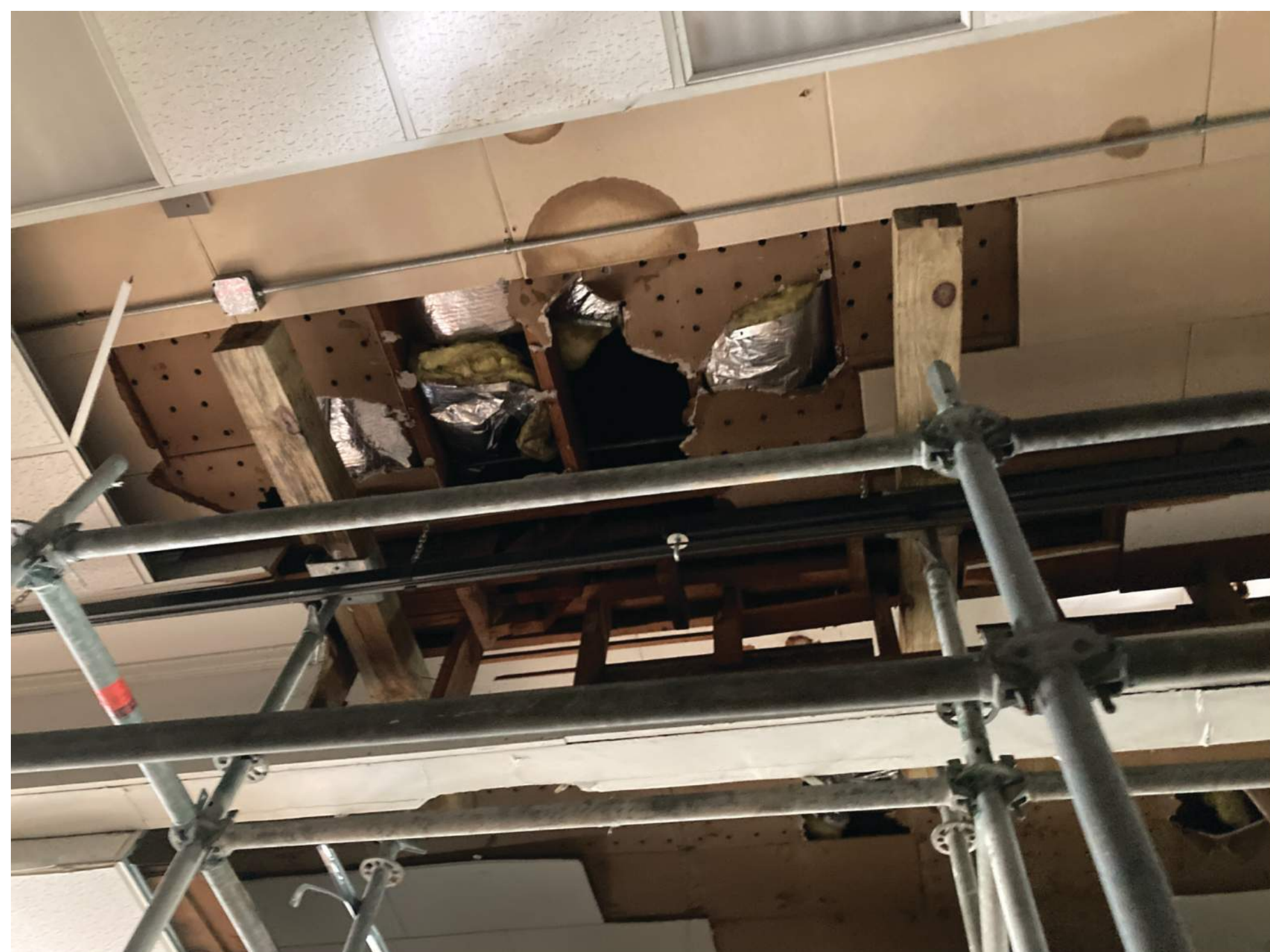
1 CEILING ABOVE THE STAGE, FIRST FLOOR
