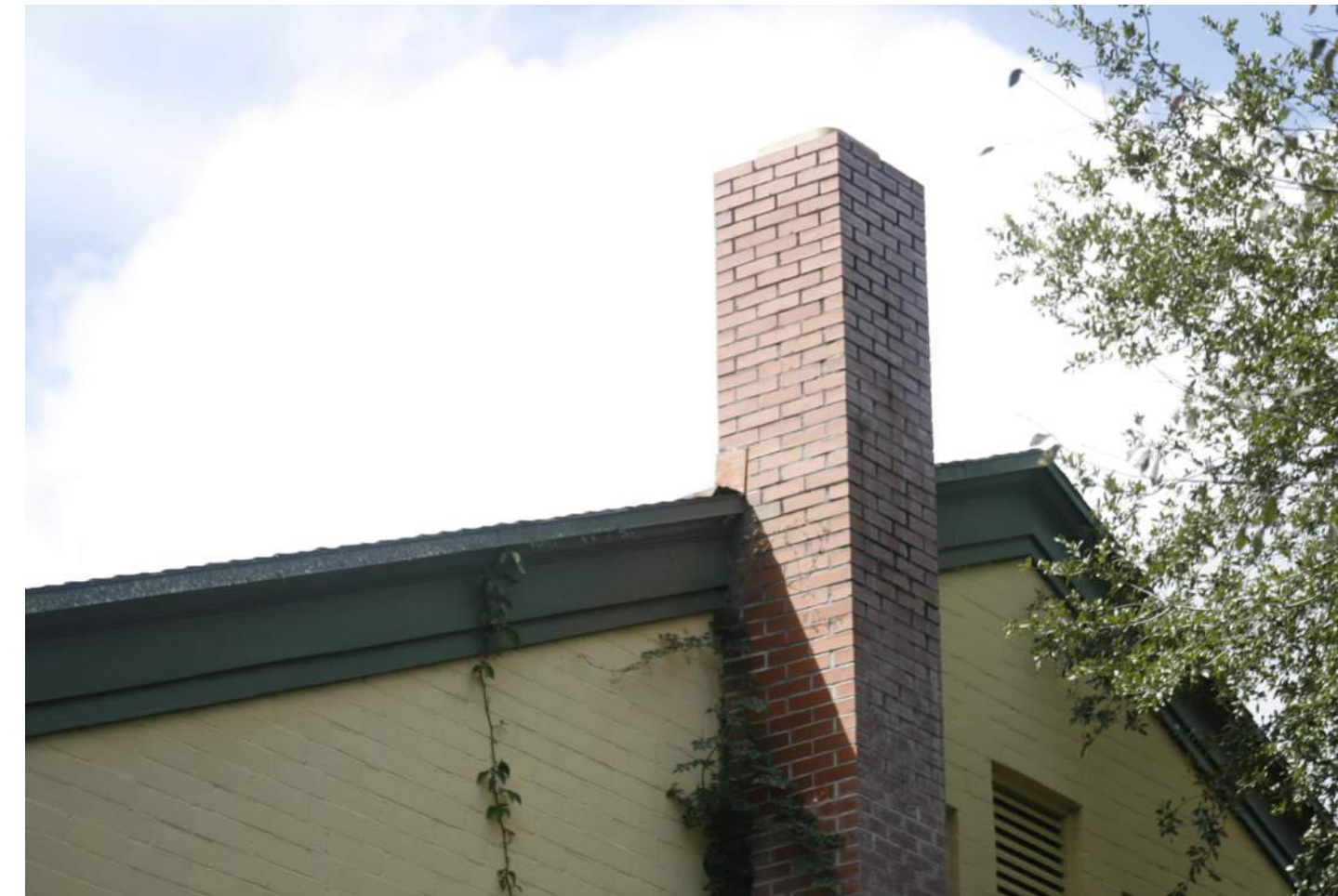
1 CHIMNEY AT NORTH
