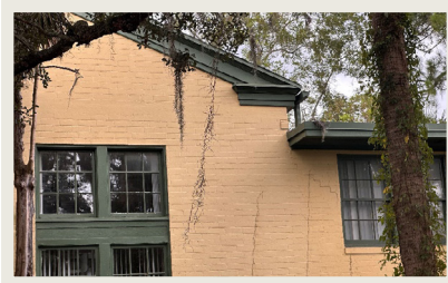
Figure 5: South Wall of Existing Auditorium
