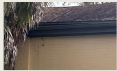
Figure 6: West Wall of Existing Auditorium
