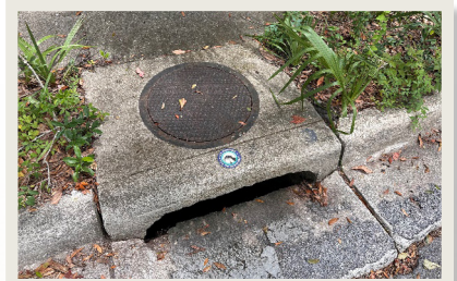
Figure 10: Existing Storm System Inlet on NE 5th St
