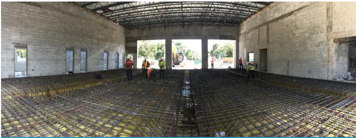
KL provides extra attention to the apparatus bay substrate construction to ensure a long-lasting floor is built to withstand the weight of current and future trucks.
