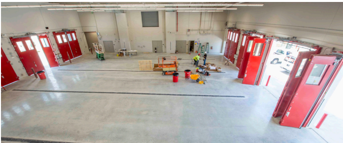
BUILDING ENHANCED APRON SLABS: RIVIERA BEACH FIRE STATION #88 As part of our Building Better Buildings program, KL offered to enhance the fire apparatus bay slab by strengthening the original 6-inch concept. The team coordinated a 4:00 AM slab pour to achieve an 8-inch slab with 2 mats of rebar in it to reinforce the slab itself. Of our own accord, we added this enhancement after researching the specs on the 54,000 lb fire trucks to ensure the optimum strength of the slab.
