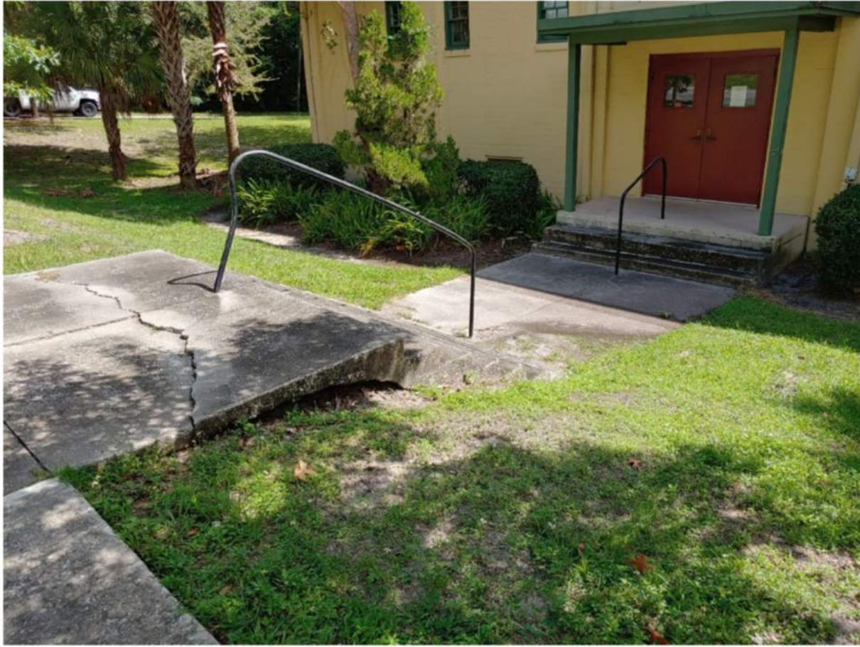
Figure 2. Stairway Undermining
