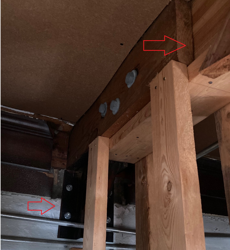
Figure 6. Retrofit seat and repaired (spliced) truss chord at south truss
