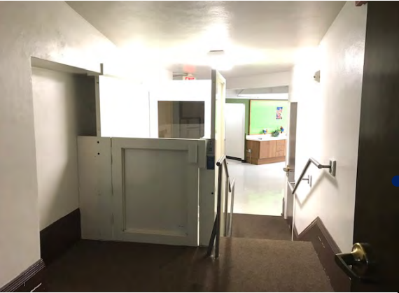
View from Main Hall to Lobby
