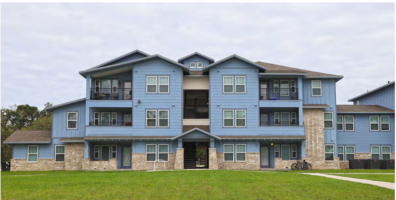
Gainesville Housing Authority: Woodland Park Phase I
