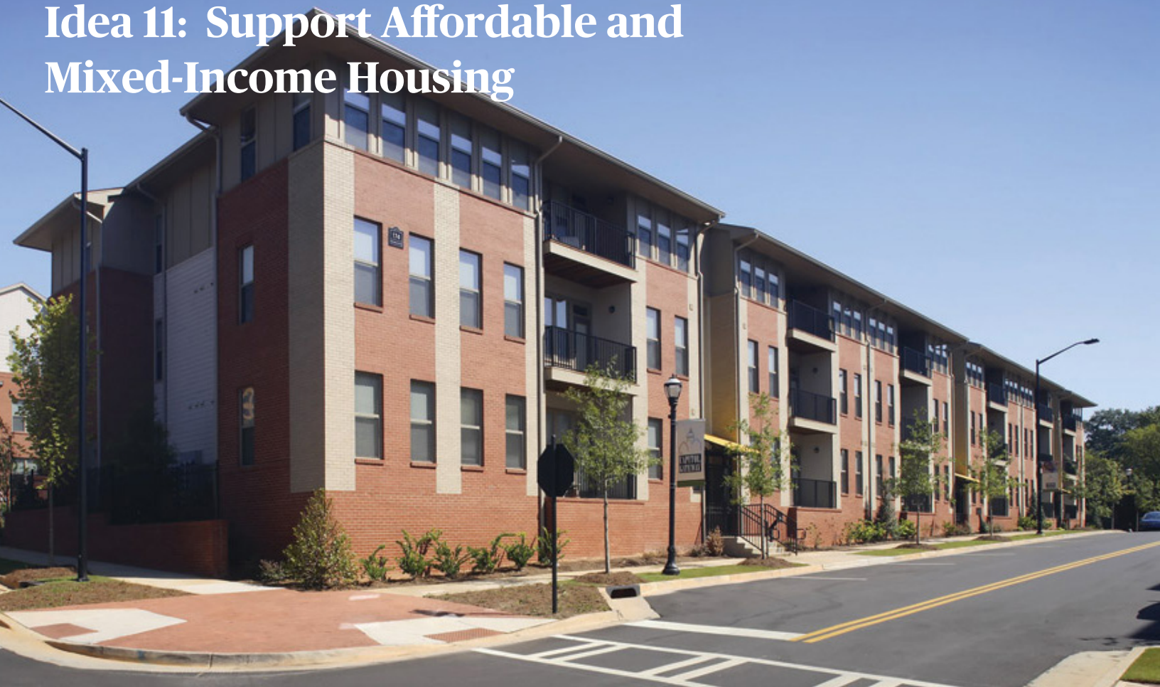
Capitol Gateway, a mixed-income development in Atlanta, GA (Source: Apartment Ratings)
