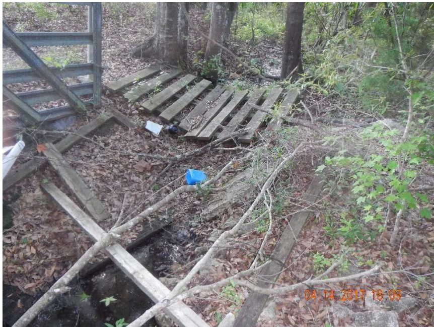
Photo 536. View of collapsed culvert and roadway at offsite drainage divide as seen looking west from GPS location 10304 (Frame 1451; 04/14/17).
