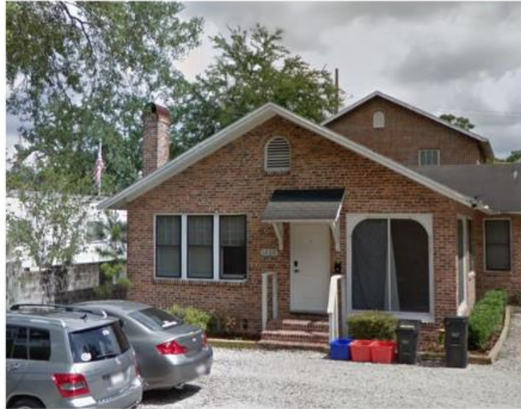
Photo 13. 1022 SW 1 st AVE, Contributing Structure in the District
