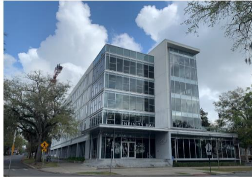
Photo 17. Oblique view of Infinity Hall, a 5-story structure, looking north.
