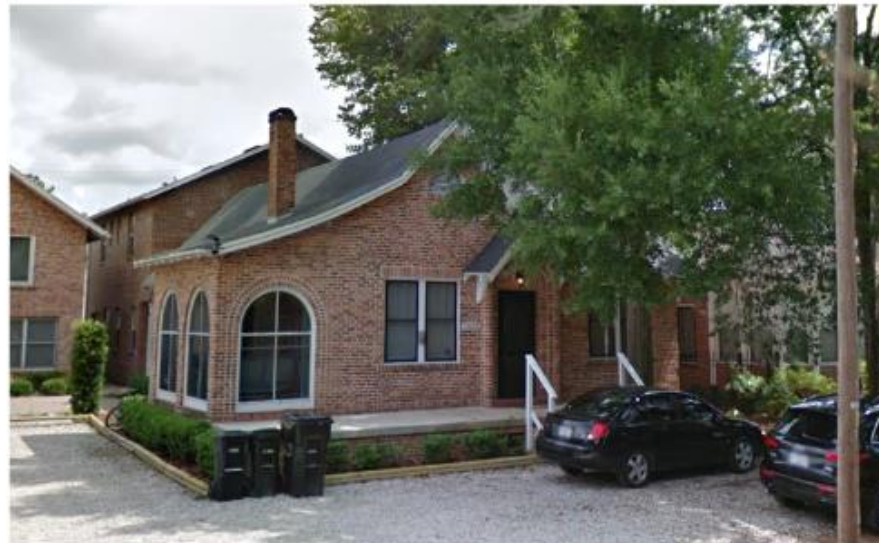
Photo 12. 1022 SW 1 st AVE, Contributing Structure in the District
