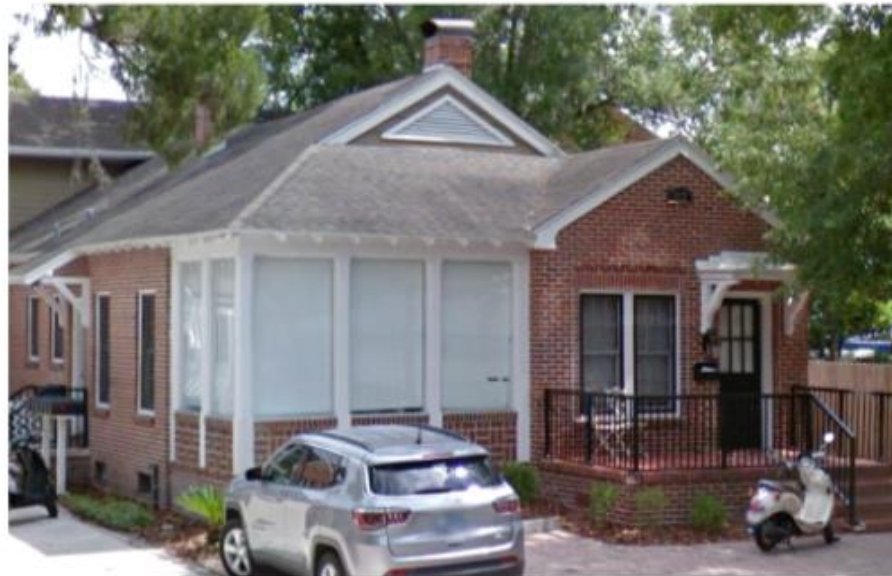
Photo 10. 1012 SW 1 st AVE, Contributing Structure in the District
