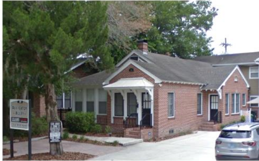
Photo 11. 1016 SW 1 st AVE, Contributing Structure in the District
