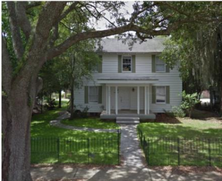
Photo 14. 1023 SW 1 st AVE, Contributing Structure in the District
