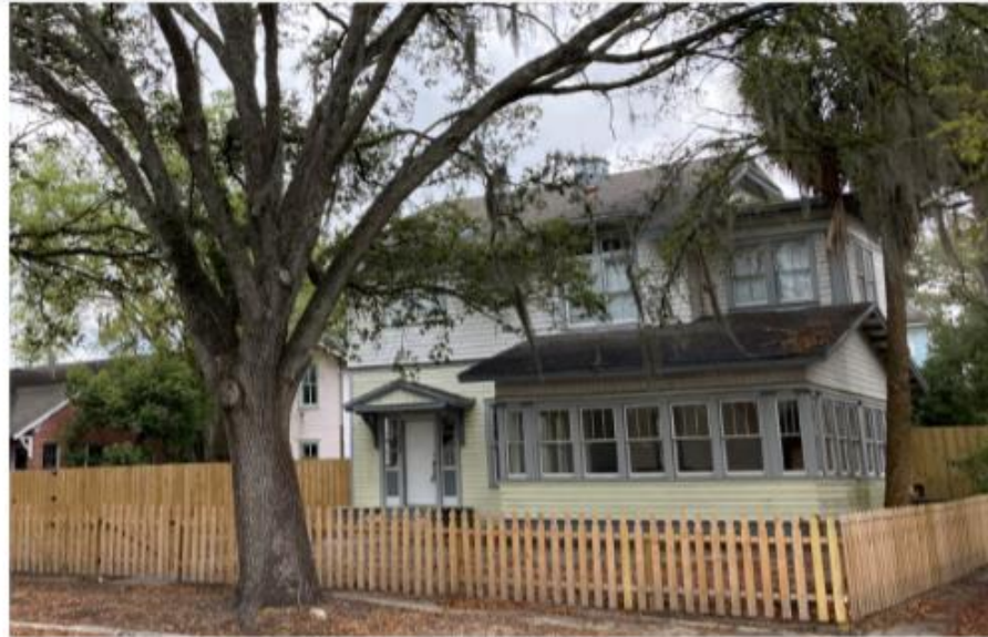
Photo 9. 1004 SW 1 st AVE, Contributing Structure in the District
