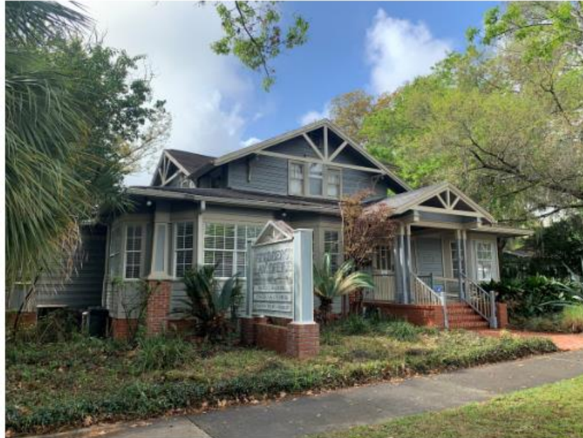
Photo 6. 1013 SW 2 nd AVE, Contributing Structure in the District
