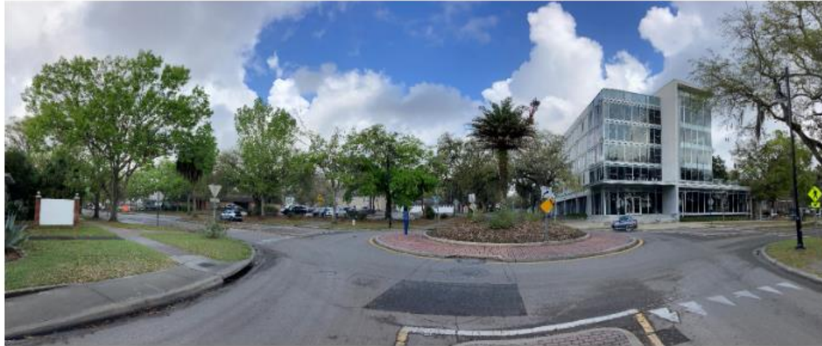
Photo 15. The intersection (roundabout) at SW 2 nd Avenue and SW 10 th Street, looking north. The proposed project would be to the top left of the photo. To the top right, is Infinity Hall, a 5-story structure.
