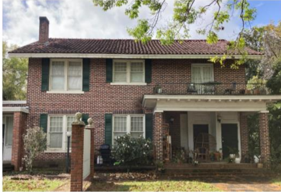
Photo 7. 1005 SW 2 nd AVE, Contributing Structure in the District
