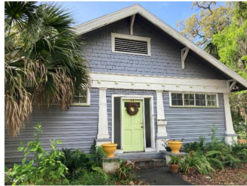
Photo 2. 1113 SW 2 nd AVE, Contributing Structure in the District
