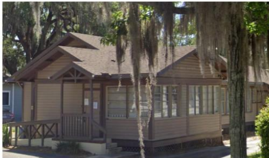
Photo 4. 1103 SW 2 nd AVE, Contributing Structure in the District
