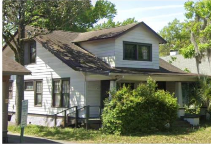
Photo 3. 1107 SW 2 nd AVE, Contributing Structure in the District
