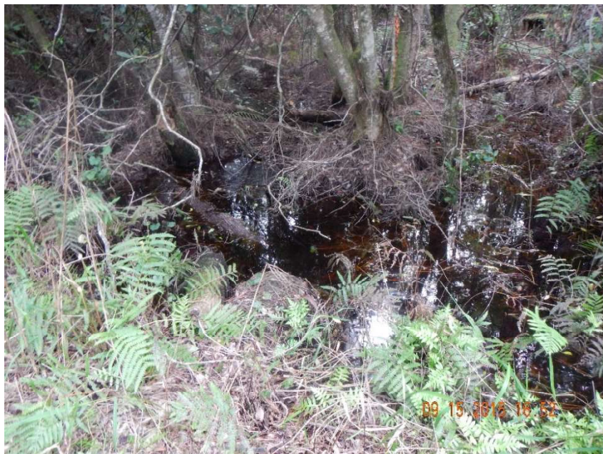
Photo 374. View of Wetland: Cypress-Mixed Hardwoods-Bays from Physical Feature: Culvert as seen looking at west end (upstream) of culvert at GPS location 7360 (Frame 7506; 09/15/15).
