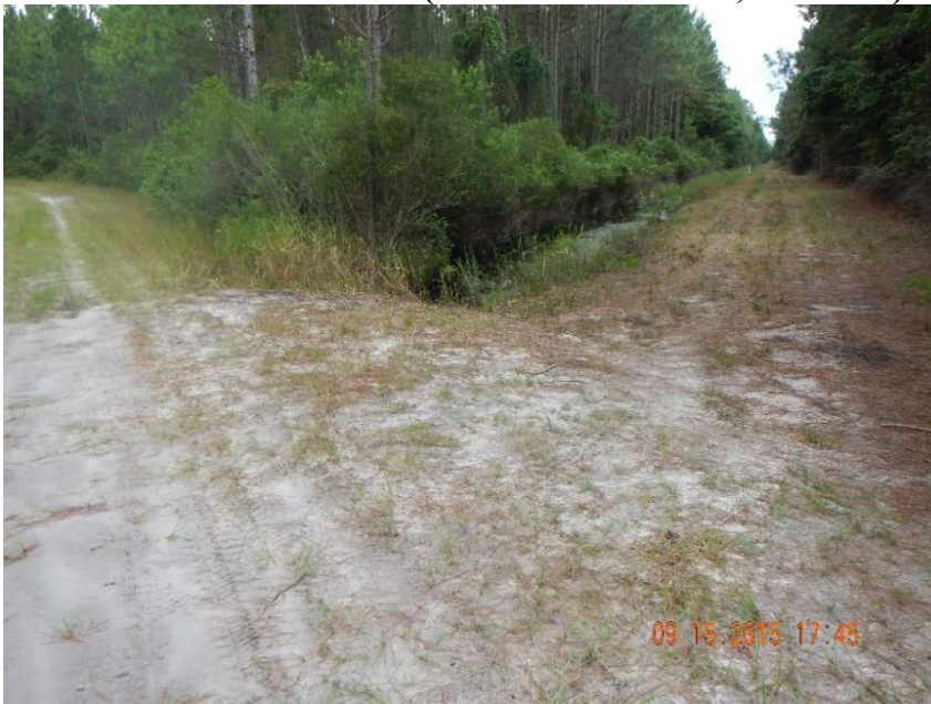
Photo 381. View of gas line (right) and forest road (left) that accesses property to the east. This photo is taken from GPS location 7403 looking southeast to south. There are several Physical Feature: Culverts at this location that route water north and east through this intersection (Frame 7515; 09/15/15).
