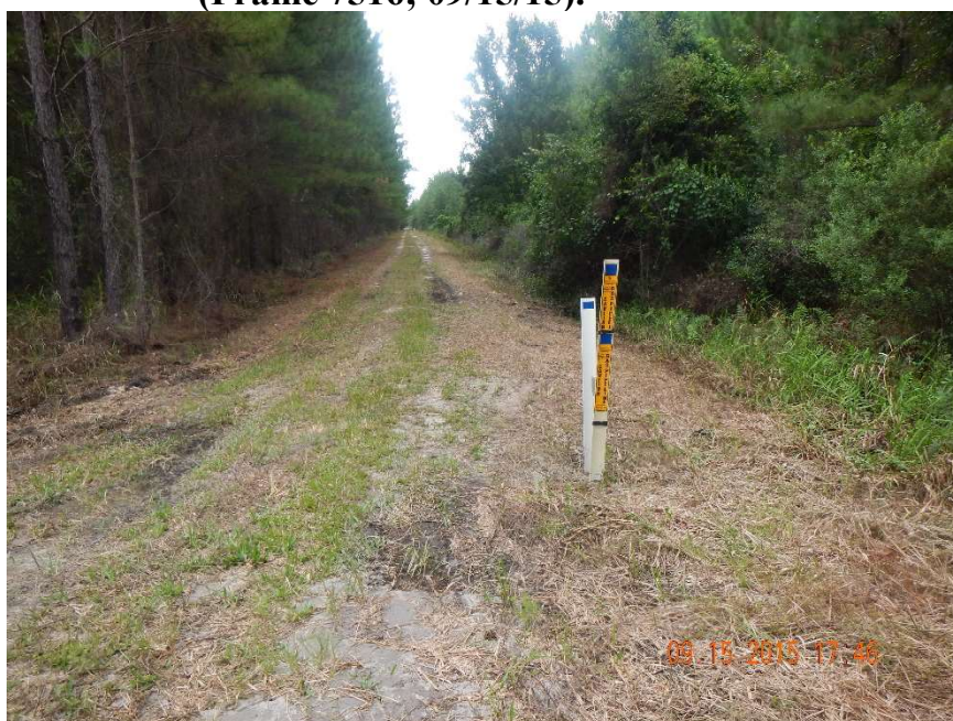
Photo 383. View to north of gas line as seen from Physical Feature: Culvert at GPS location 7404 (Frame 7517; 09/15/15).
