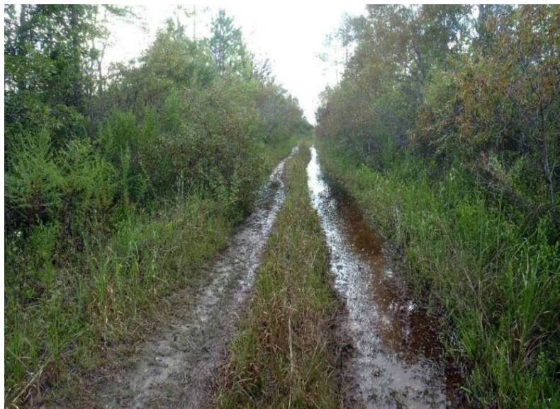
Photo 334. View of Wetland: Natural Flow-way occurring across the top of the improved forest road as seen looking northwest from GPS location 6758 (Frames 2125-2126; 09/10/15).
