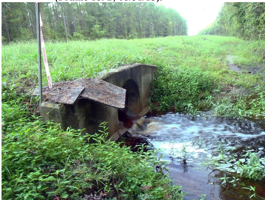
Photo 218. View of Physical Feature: Culvert located on east side of road as seen at GPS location 1697 (Frame 1893; 08/31/15).
