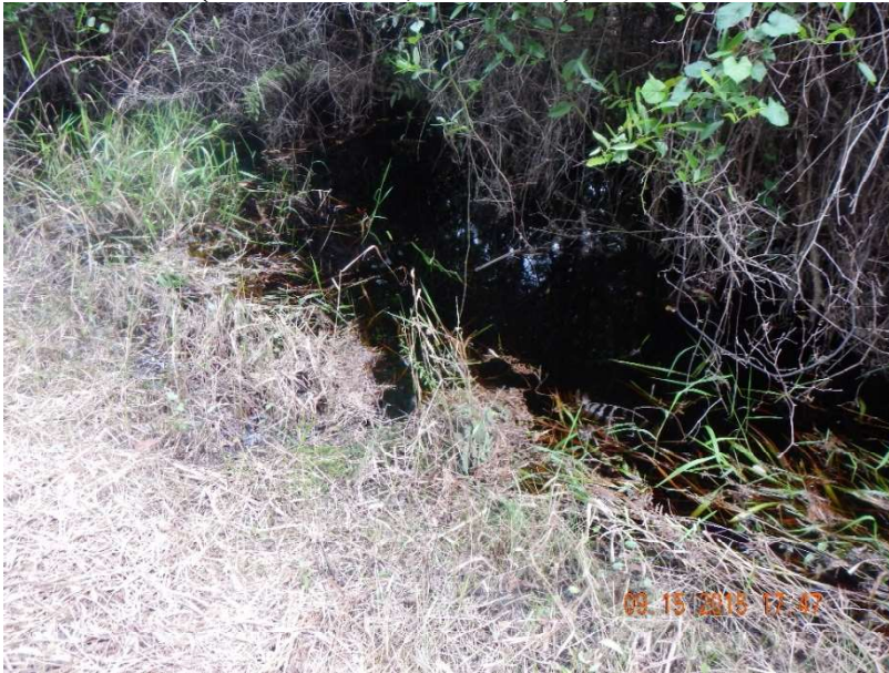
Photo 385. View of east area at east end (downstream) of Physical Feature: Culvert located at GPS location 7405. Water flows here from GRU property, north into ditch along gas line, then east into a large wetland area (Frame 7519; 09/15/15).
