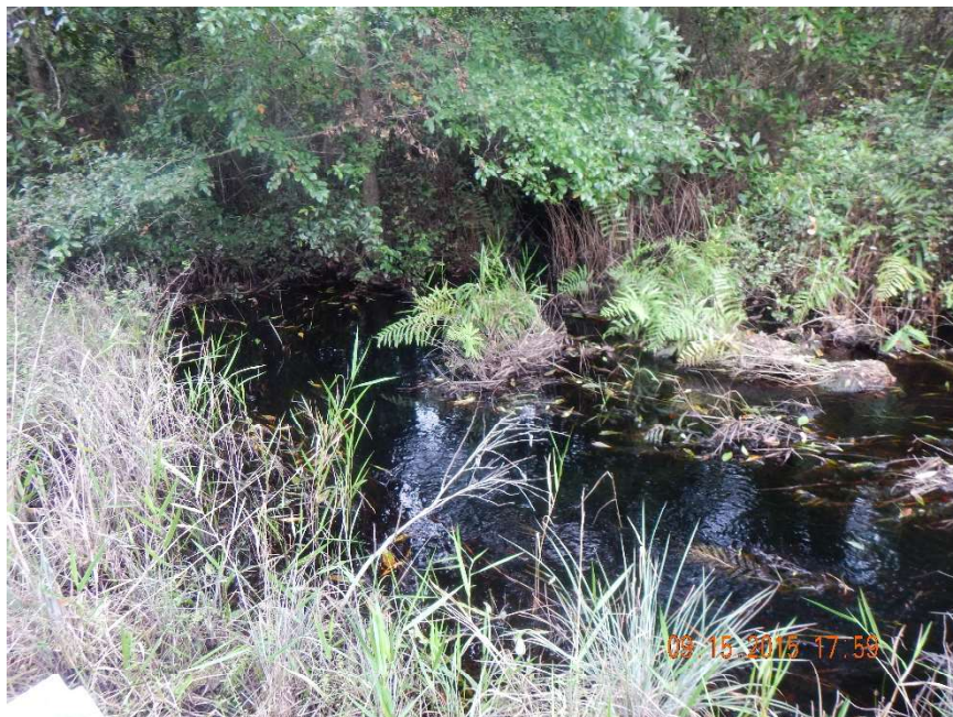
Photo 386. View of flow-way at east end of Physical Feature: Culvert located in gas line right-of-way at GPS location 7421 (Frame 7520; 09/15/15).
