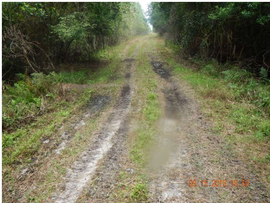
Photo 372. View to south of gas line through Wetland: Cypress-Mixed Hardwoods-Bays as seen at culvert location at GPS location 7360 (Frame 7503; 09/15/15).
