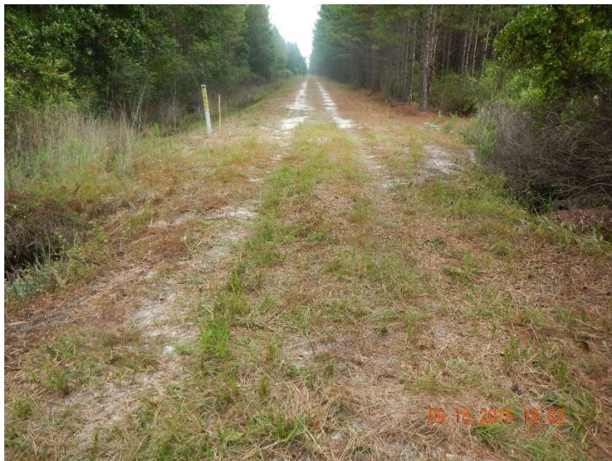
Photo 388. View of Physical Feature: Culvert area within gas line right-of-way as seen looking south from GPS location 7421 (Frame 7522; 09/15/15).
