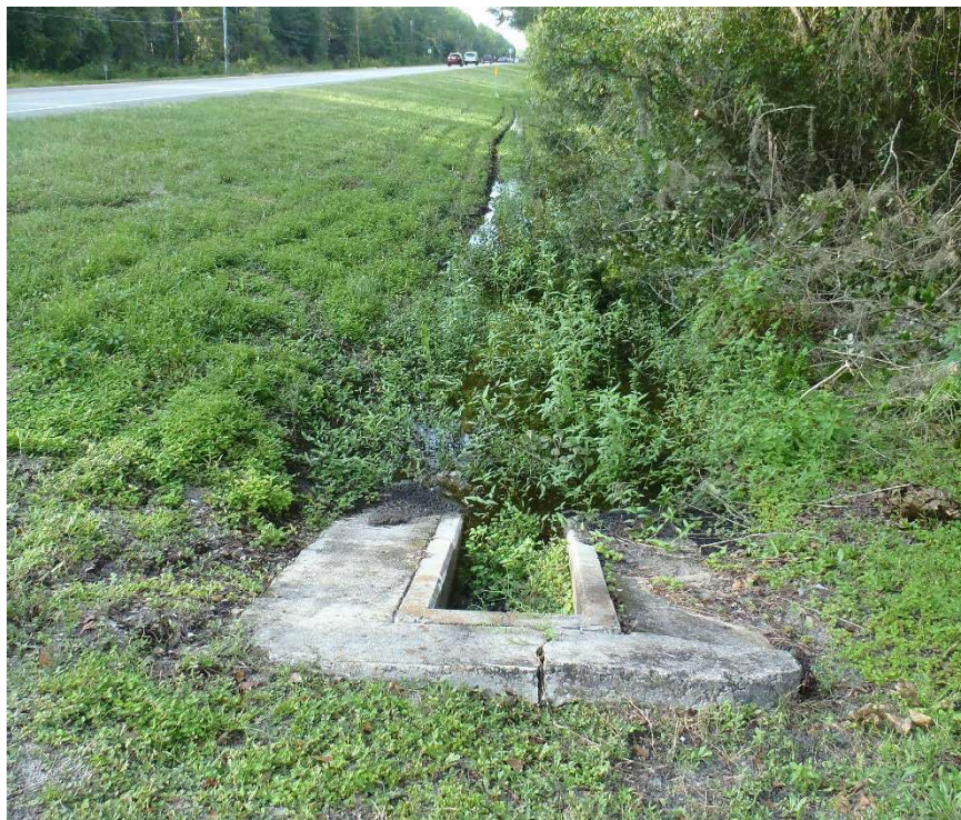
Photo 235. View of Physical Feature: Culvert located on east side of road as seen looking north from GPS location 5199 (Frame 1927; 09/02/15).
