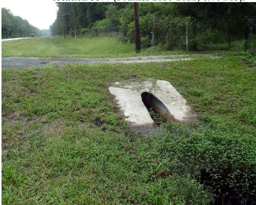
Photo 285. View of Physical Feature: Culvert as seen looking east from GPS location 5885 (Frame 2022; 09/04/15).
