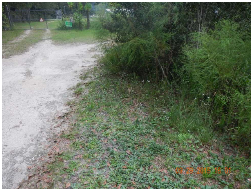
Photo 440. View of south side of Physical Feature: Culvert at GPS locations 8101-8102 (Frame 7651; 09/29/15).
