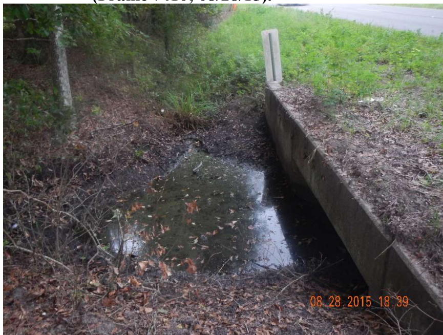
Photo 195. Rocky Creek: view to south of culverts located at GPS location 1517 on east side of CR 231 at GPS location 1517 (Frame 7411; 08/28/15).
