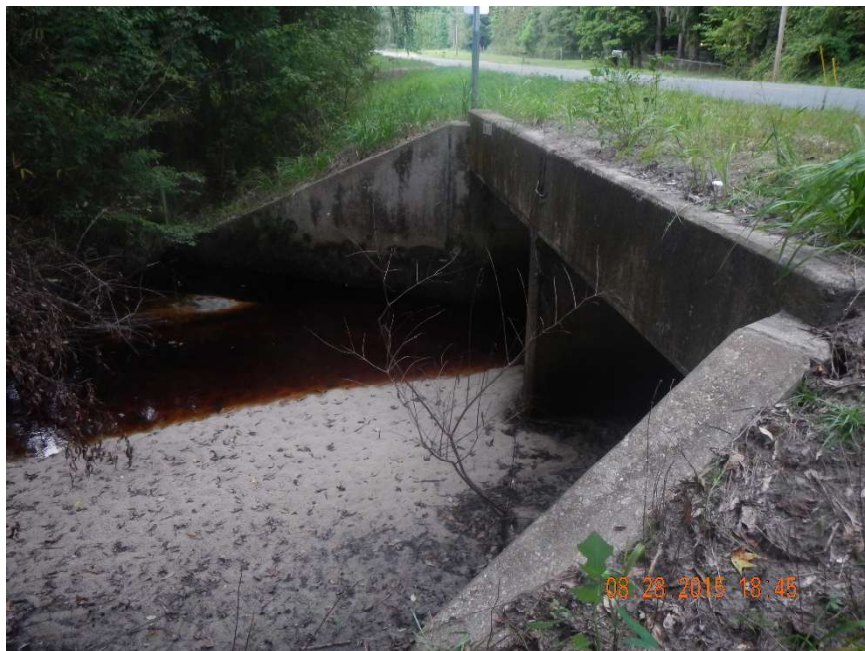
Photo 198. View to south of box culverts on east side (upstream) of CR 231 in Rocky Creek at GPS location 1518 (Frame 7416; 08/28/15).
