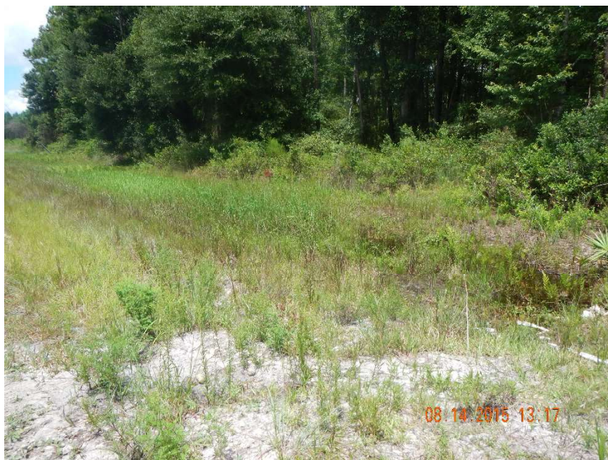
Photo 2. Power line ditch located at GPS location 4 (Frame 7356; 08/14/15).
