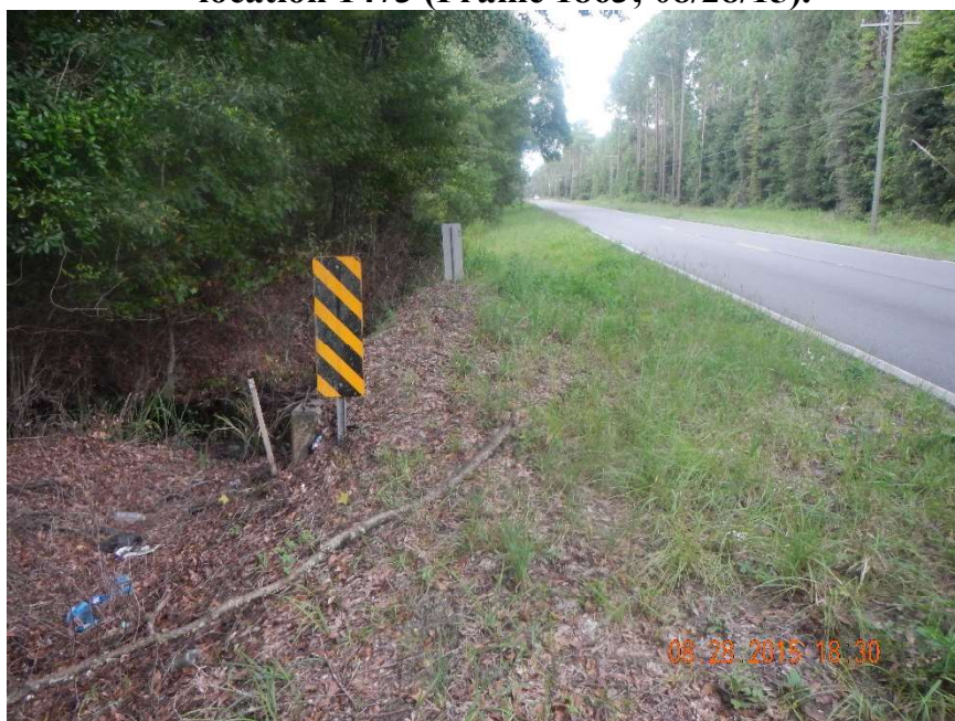
Photo 191. Rocky Creek: view to south of east side of culverts at CR 231 at GPS location 1516 (Frame 7406; 08/28/15).
