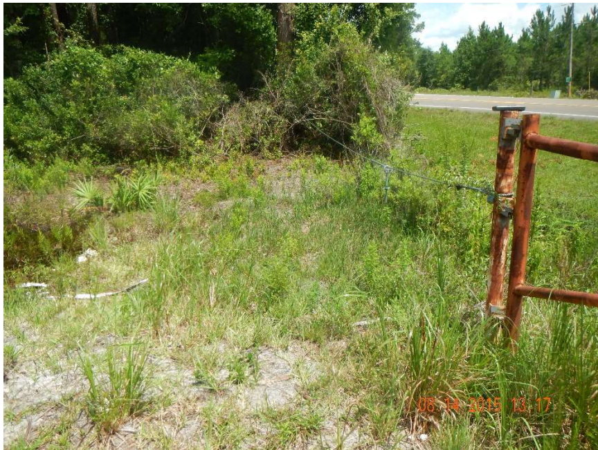
Photo 1. Berm located at GPS location 4 (Frame 7355; 08/14/15).
