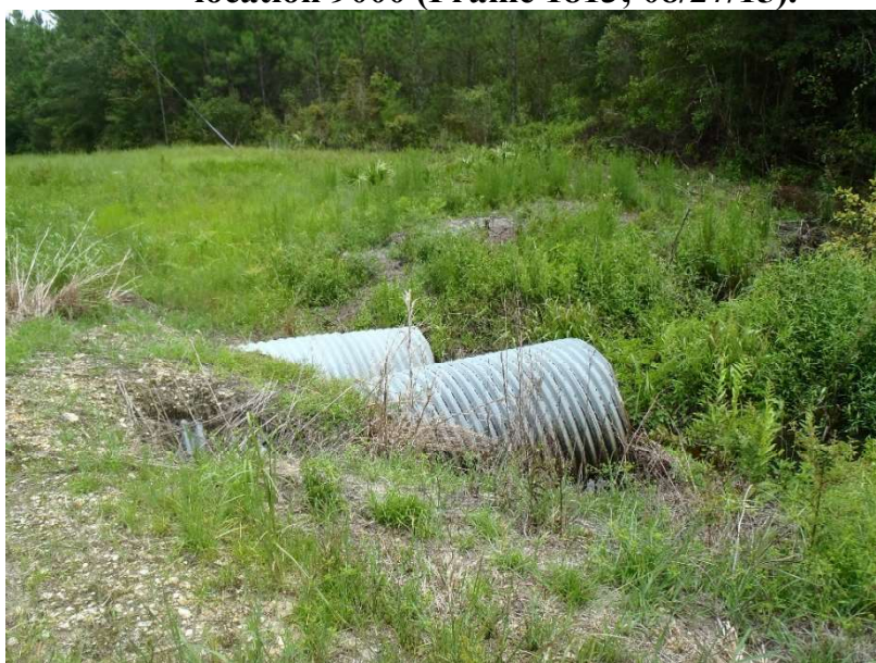
Photo 161. View of culverts on south side of power line easement within the Planted Pine-Mesic Pine Flatwoods located at GPS location 9000 (Frame 1814; 08/27/15).
