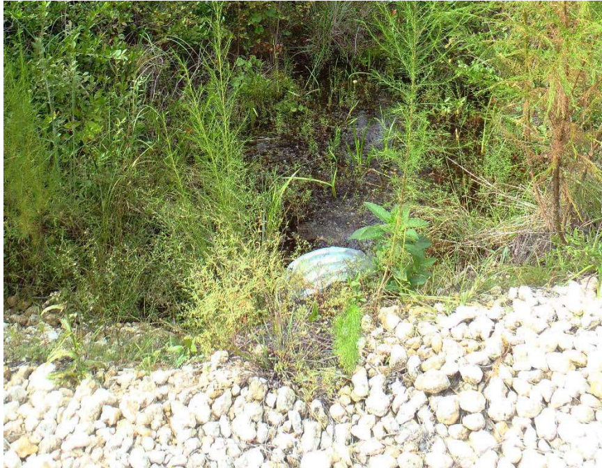
Photo 174. View of Physical Feature: Culvert located on north side of road at GPS location 1272 (Frame 1835; 08/27/15).
