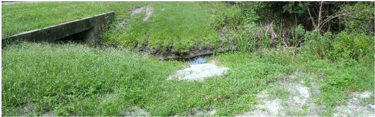
Photo 145. View of Physical Feature: Culvert as seen looking north from GPS location 1040 (Frames 1785-1786; 08/26/15).
