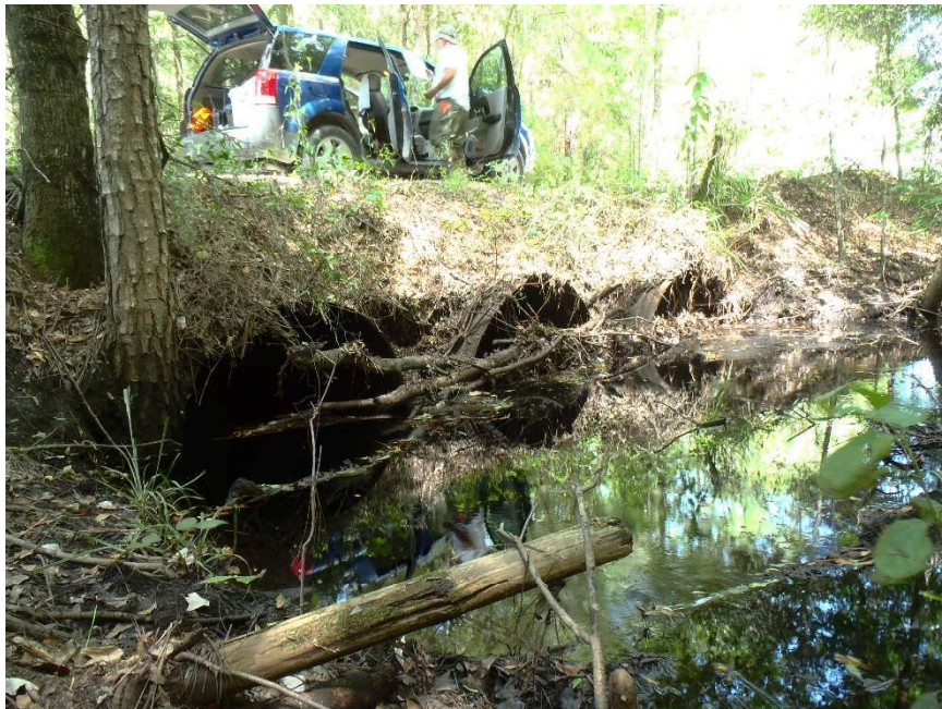
Photo 23. View of three culverts as seen at GPS location 9 (Frame 1490; 08/14/15).
