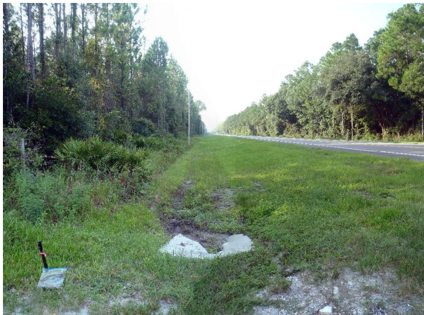
Photo 117. View of Physical Feature: Culvert as seen looking north from GPS location 2276 (Frames 1725-1726; 08/25/15).
