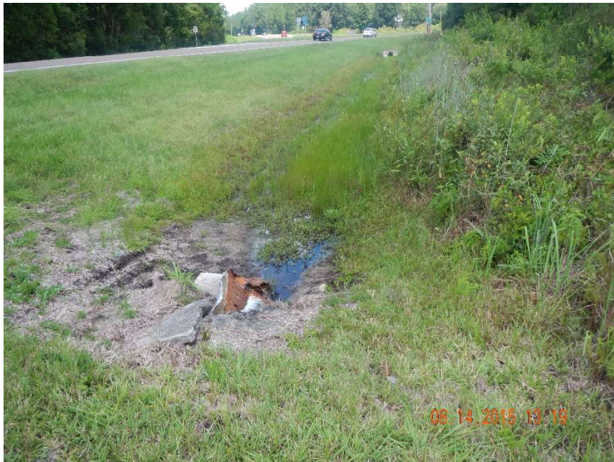
Photo 9. Culvert and ditch located on north side of GPS location 1 (Frame 7363; 08/14/15).
