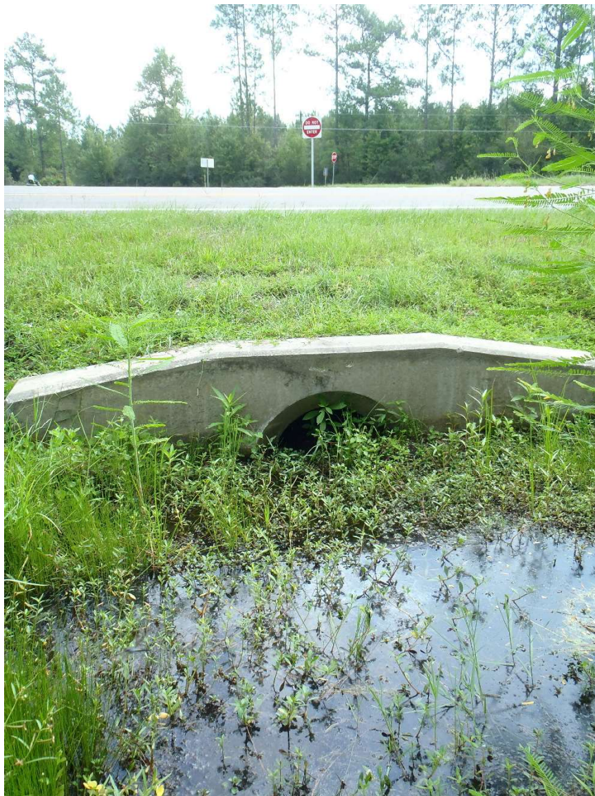
Photo 127. View of Physical Feature: Culvert at GPS location 2340 (Frame 1745; 08/26/15).
