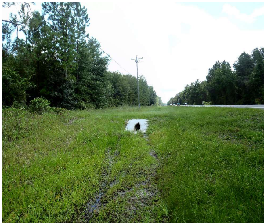
Photo 143. View of Physical Feature: Culvert as seen looking south from GPS location 1038 (Frames 1781-1782; 08/26/15).
