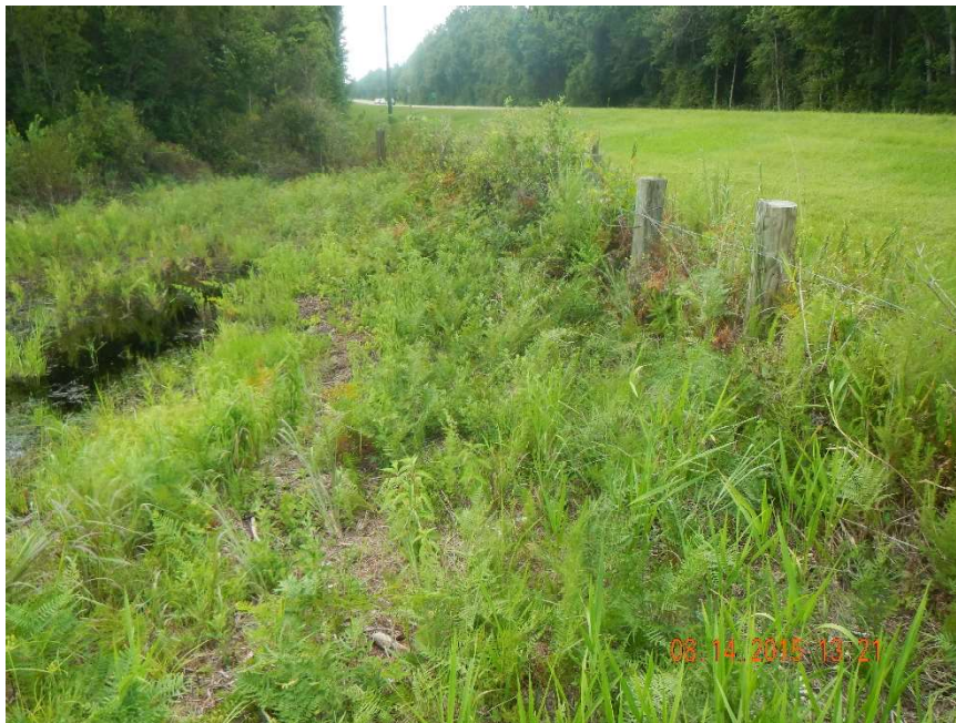
Photo 10. Berm (ditch block) located at GPS location 5 as seen looking south (Frame 7364; 08/14/15).
