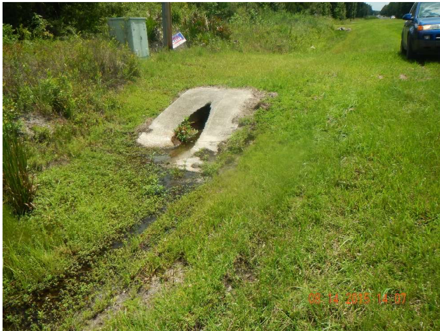
Photo 15. Culvert as seen looking south from GPS location 7 (Frame 7369; 08/14/15).
