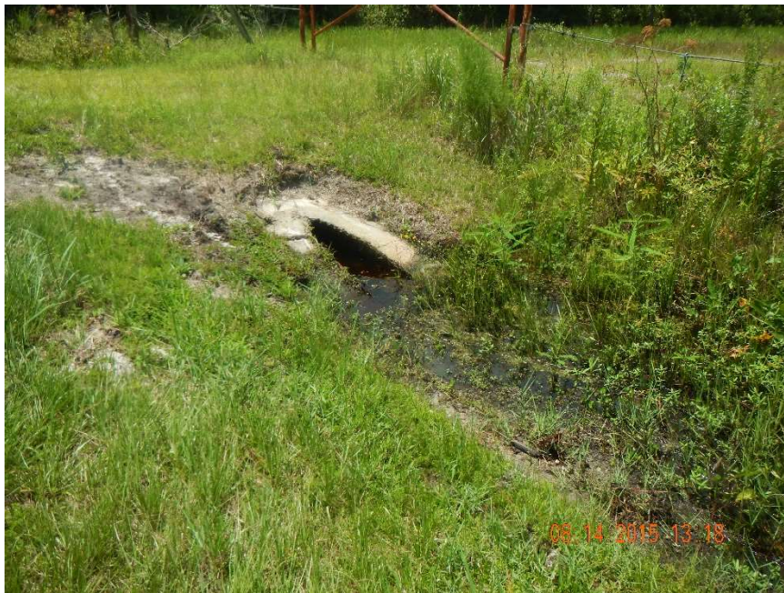
Photo 6. Culvert located on south side of GPS location 2 (Frame 7360; 08/14/15).
