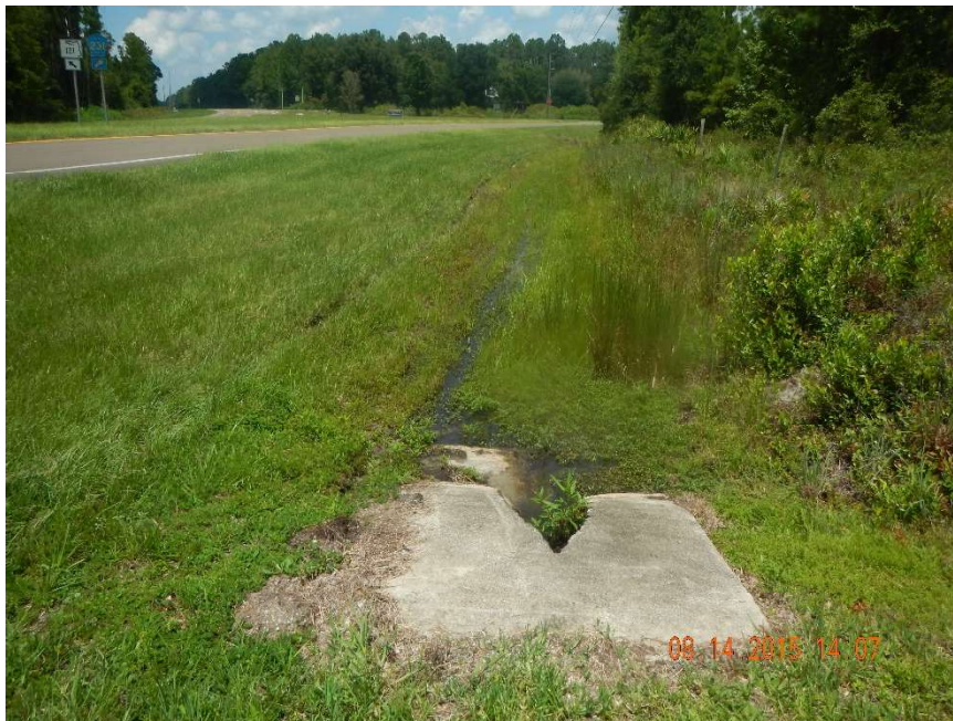
Photo 16. Culvert and ditch as seen looking north from GPS location 7 (Frame 7370; 08/14/15).
