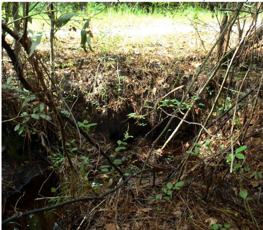
Photo 177. View of Physical Feature: Culvert located on south side of road at GPS location 1308 (Frame 1840; 08/27/15).
