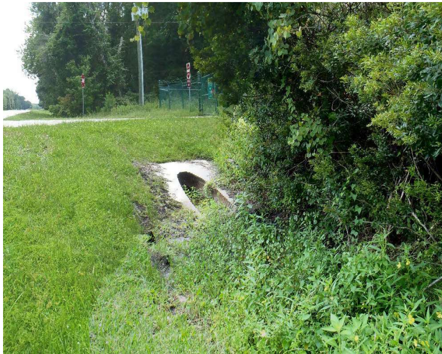
Photo 139. View of Physical Feature: Culvert as seen looking south from GPS location 1032 (Frames 1771-1772; 08/26/15).
