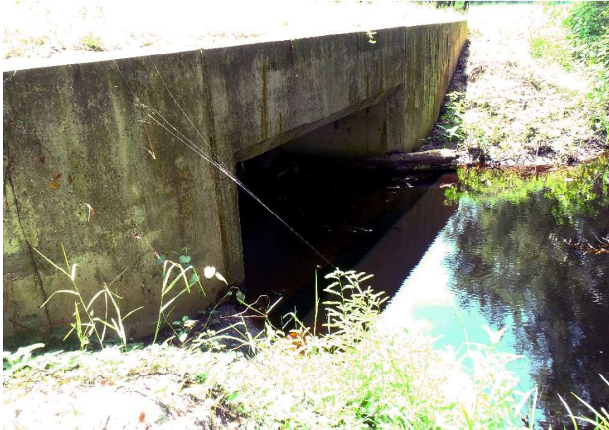
Photo 130. View of Physical Feature: Culvert at GPS location 2344 (Frame 1750; 08/26/15).
