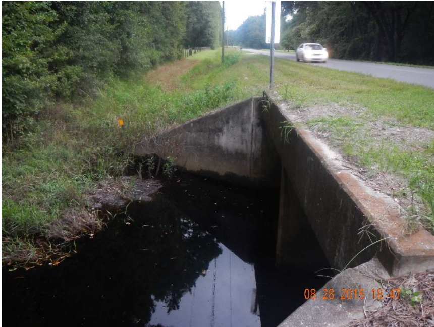
Photo 200. Rocky Creek: view to north along CR 231 of west side of box culverts located at GPS location 1518 (Frame 7420; 08/28/15).
