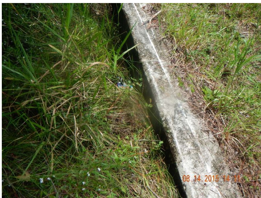
Photo 18. Culvert headwall at GPS location 8 (Frame 7372; 08/14/15).
