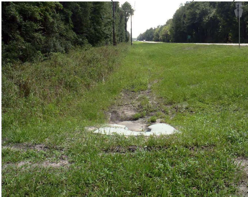
Photo 146. View of Physical Feature: Culvert as seen looking south from GPS location 1040 (Frame 1787; 08/26/15).
