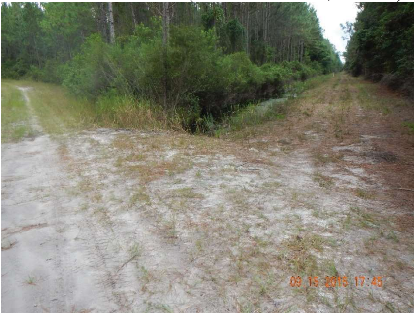
Photo 381. View of gas line (right) and forest road (left) that accesses property to the east. This photo is taken from GPS location 7403 looking southeast to south. There are several Physical Feature: Culverts at this location that route water north and east through this intersection (Frame 7515; 09/15/15).
