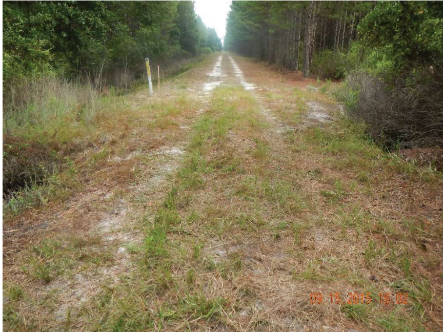
Photo 388. View of Physical Feature: Culvert area within gas line right-of-way as seen looking south from GPS location 7421 (Frame 7522; 09/15/15).
