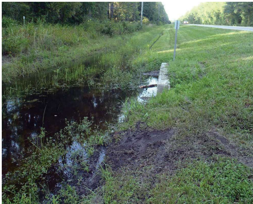
Photo 237. View of Physical Feature: Culvert located on west side of road as seen looking north from GPS location 5201 (Frame 1929; 09/02/15).
