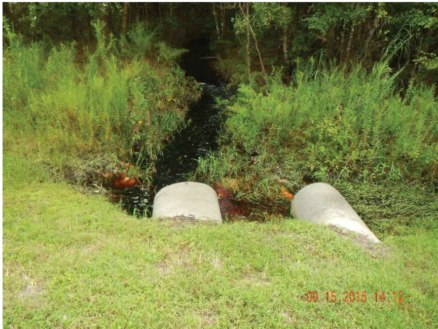
Photo 360. View to south (upstream) of culverts located in Rocky Creek at GPS location 9841 (Frame 7490; 09/15/15).
