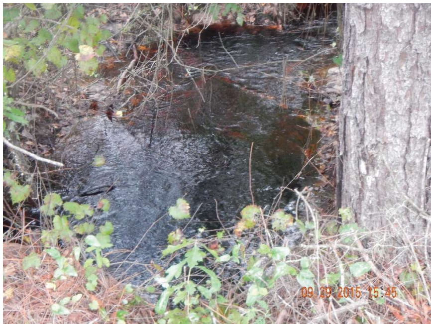
Photo 438. View of flow at Physical Feature: Culvert at GPS location 8100. Flow is to north on north side of road (Frame 7649; 09/29/15).
