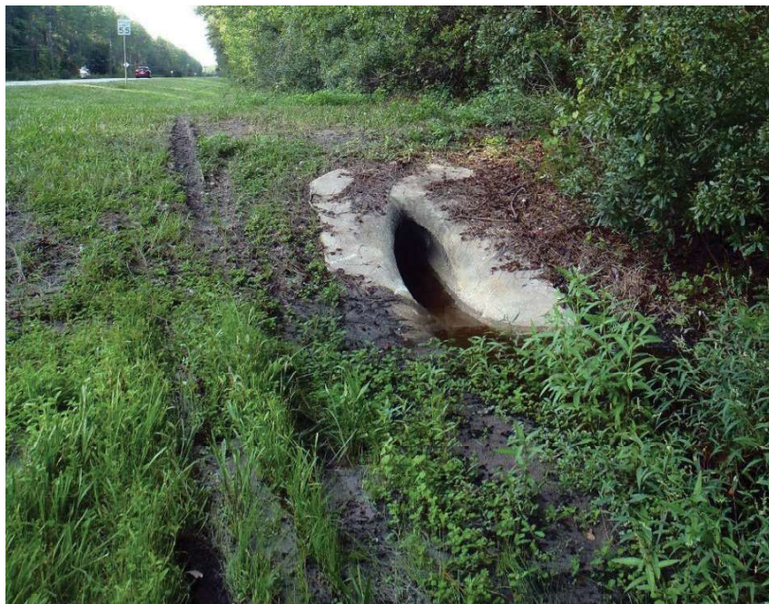
Photo 239. View of Physical Feature: Culvert located on east side of road as seen looking north from GPS location 5203 (Frame 1931; 09/02/15).
