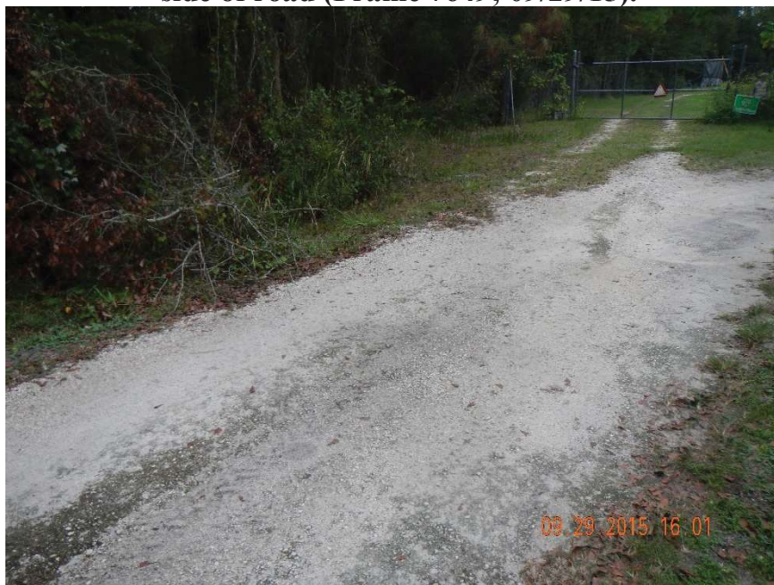
Photo 439. View of Physical Feature: Culvert at GPS locations 8101-8102. View is of north side of culvert (Frame 7650; 09/29/15).
