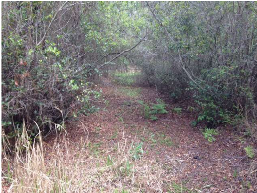
Photo 555. View of excavated ditch located at GPS location 10407 (Frame 592; 04/18/17).
