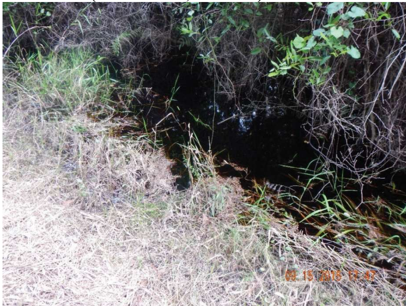
Photo 385. View of east area at east end (downstream) of Physical Feature: Culvert located at GPS location 7405. Water flows here from GRU property, north into ditch along gas line, then east into a large wetland area (Frame 7519; 09/15/15).
