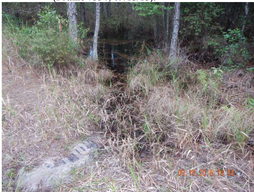
Photo 399. View of Physical Feature: Culvert as seen looking north (downstream) from GPS location 7497 (Frame 7535; 09/15/15).
