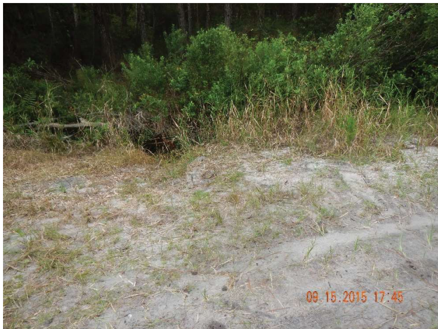
Photo 382. View of north end of Physical Feature: Culvert that runs north from GPS location 7403 to 7404 and routes water in this direction (Frame 7516; 09/15/15).
