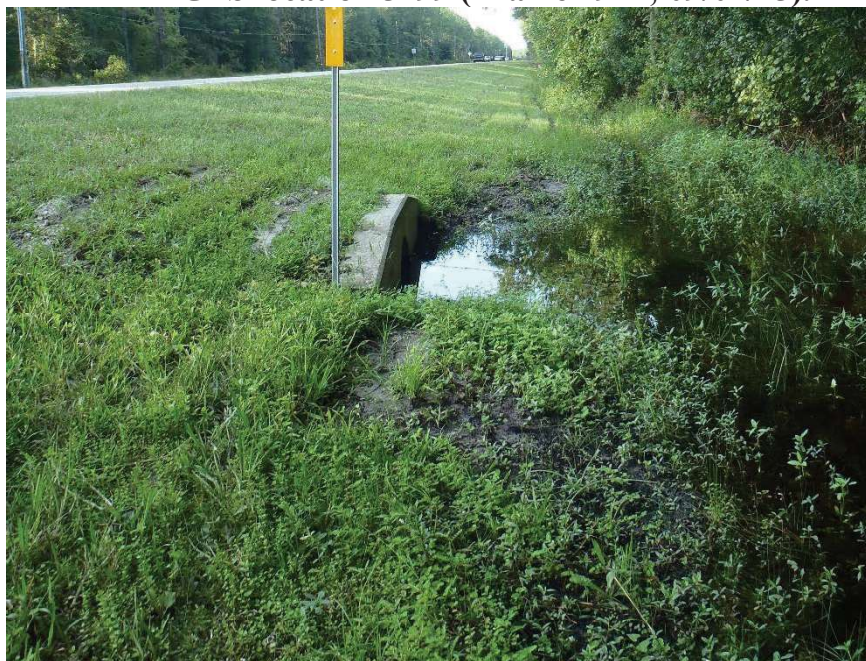
Photo 236. View of Physical Feature: Culvert located on east side of road as seen looking north from GPS location 5200 (Frame 1928; 09/02/15).
