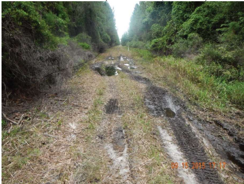
Photo 379. View of gas line as seen looking north from GPS location 7378 Wetland: Natural Flowway, which occurs from west to east across top of gas line extending from GPS locations 7375–7380 (Frame 7512 (09/15/15).
