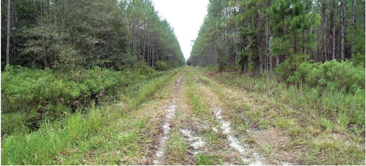
Photo 410. View of flow-way across top of gas line access road as seen looking south from GPS location 7756. Flow-way extends from GPS location 7756 south to 7757, a distance of 325 ft (Frames 2183-2184; 09/18/15).
