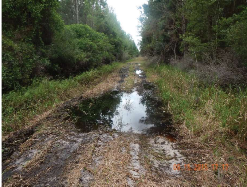
Photo 378. View of gas line as seen looking south from GPS location 7378 Wetland: Natural Flowway, which occurs from west to east across top of gas line extending from GPS locations 7375–7380 (Frame 7511; 09/15/15).
