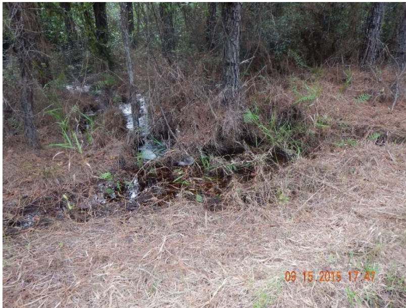
Photo 384. View of area at west end of Physical Feature: Culvert located at GPS location 7405. This is upstream area west of gas line (Frame 7518; 09/15/15).
