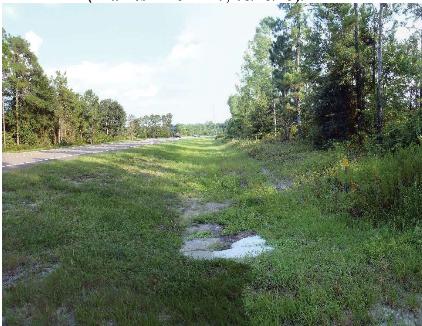
Photo 118. View of Physical Feature: Culvert as seen looking south from GPS location 2276 (Frames 1727-1728; 08/25/15).
