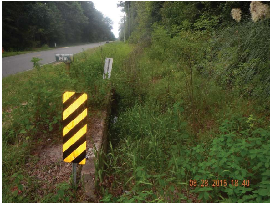
Photo 196. Rocky Creek: view to south of culvert at west side of CR 231 at GPS location 1517 (Frame 7412; 08/28/15).
