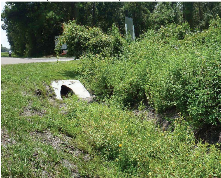
Photo 140. View of Physical Feature: Culvert as seen looking south from GPS location 1033 (Frames 1773-1774; 08/26/15).
