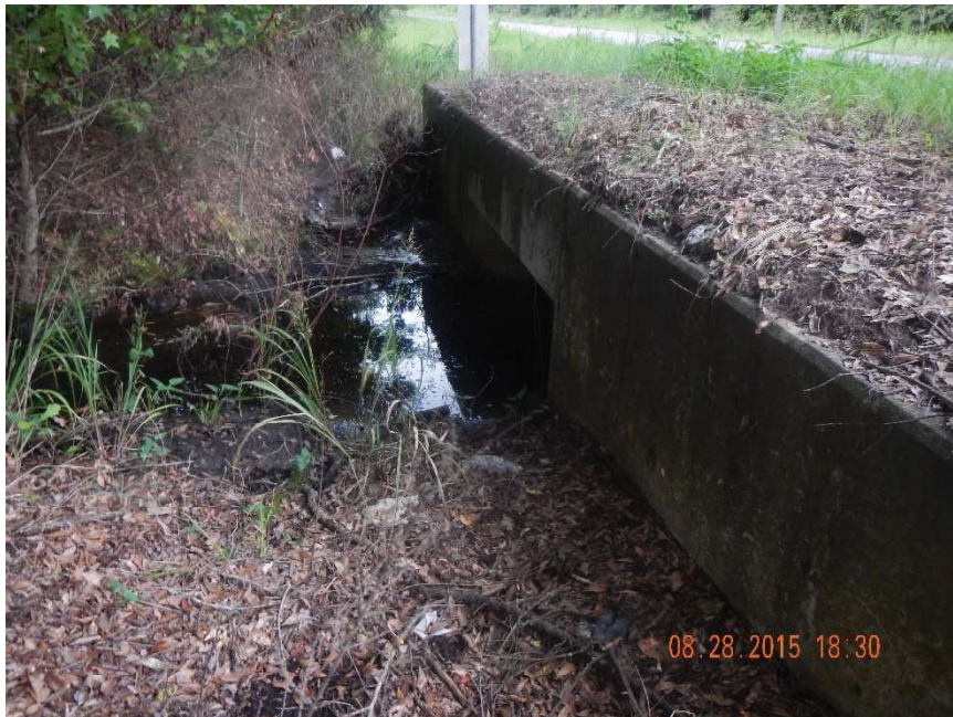
Photo 192. Rocky Creek: view to south of box culvert on east side CR 231 at GPS location 1516 (Frame 7407; 08/28/15).
