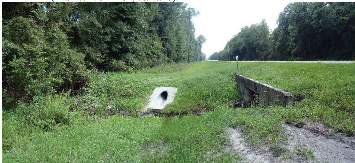
Photo 144. View of Physical Feature: Culvert as seen looking south from GPS location 1039 (Frames 1783-1784; 08/26/15).
