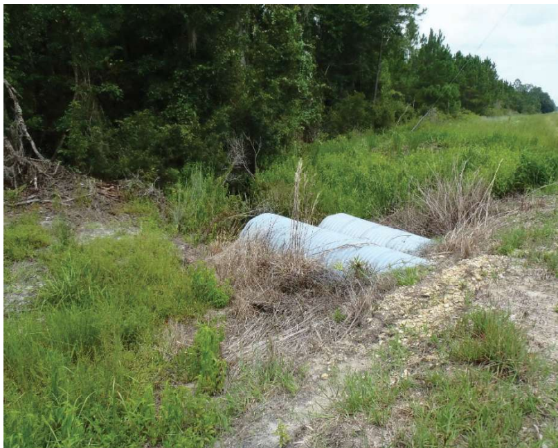
Photo 160. View of culverts on north side of power line easement within the Planted Pine-Mesic Pine Flatwoods located at GPS location 9000 (Frame 1813; 08/27/15).
