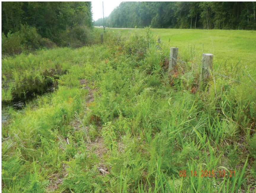
Photo 10. Berm (ditch block) located at GPS location 5 as seen looking south (Frame 7364; 08/14/15).
