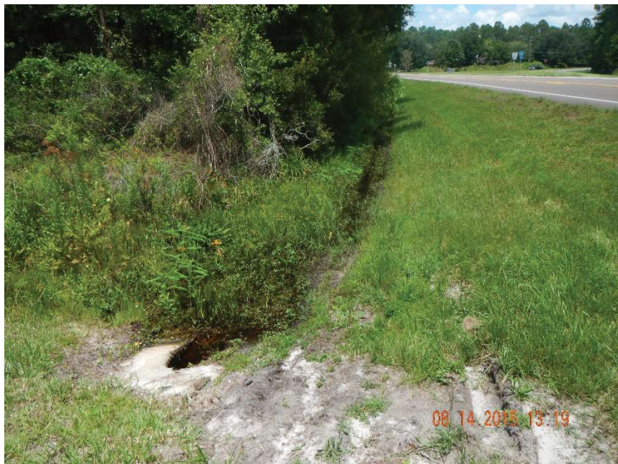
Photo 7. Culvert and ditch located on north side of GPS location 2 (Frame 7361; 08/14/15).
