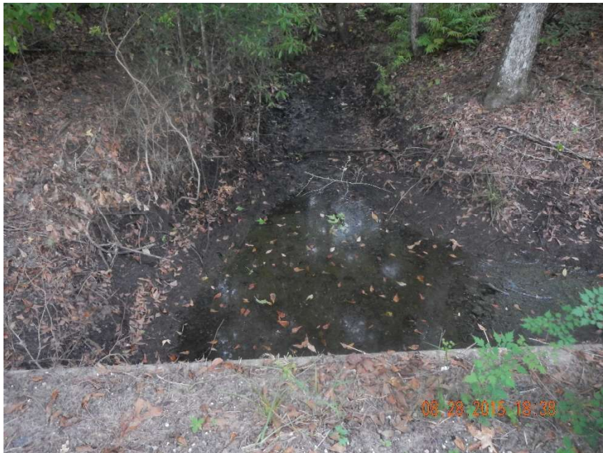
Photo 194. Rocky Creek: view to east (downstream) of CR 231 culverts located at GPS location 1517 (Frame 7410; 08/28/15).
