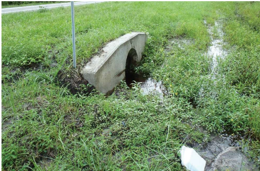
Photo 217. View of Physical Feature: Culvert located on west side of road as seen at GPS location 1696 (Frame 1892; 08/31/15).
