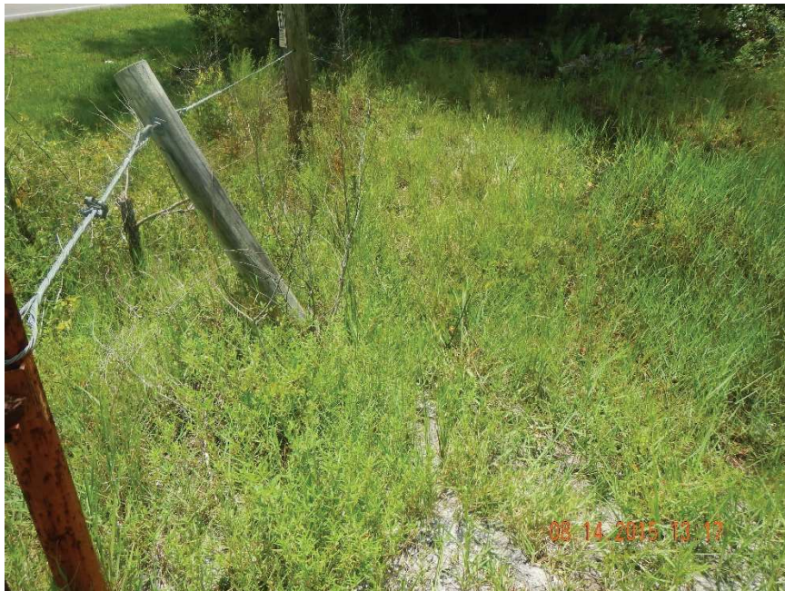
Photo 3. Berm (ditch block) located at GPS location 3 (Frame 7357; 08/14/15).
