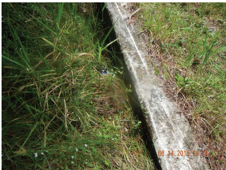
Photo 18. Culvert headwall at GPS location 8 (Frame 7372; 08/14/15).
