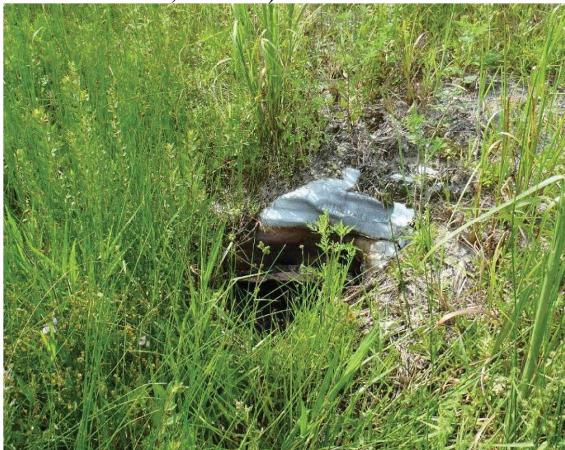
Photo 156. View of Physical Feature: Culvert located at GPS location 1117 (Frame 1806; 08/26/15).
