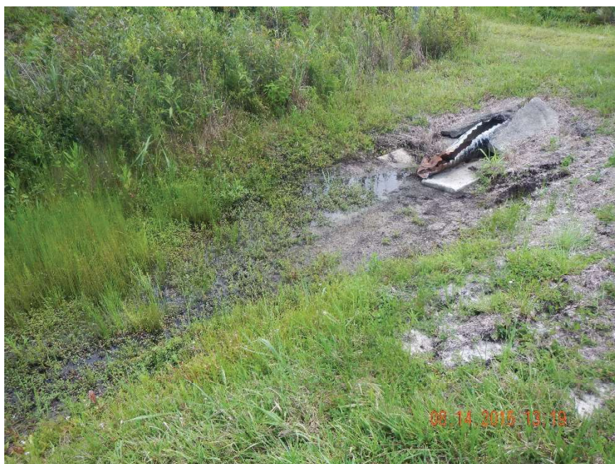
Photo 8. Culvert located on south side of GPS location 1 (Frame 7362; 08/14/15).
