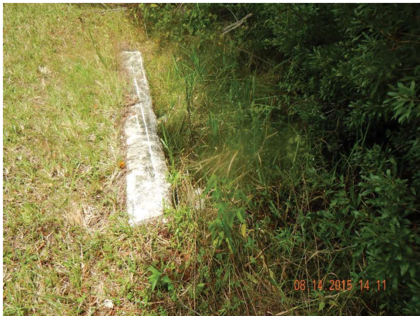
Photo 17. Culvert headwall as seen looking north from GPS location 8 (Frame 7371; 08/14/15).
