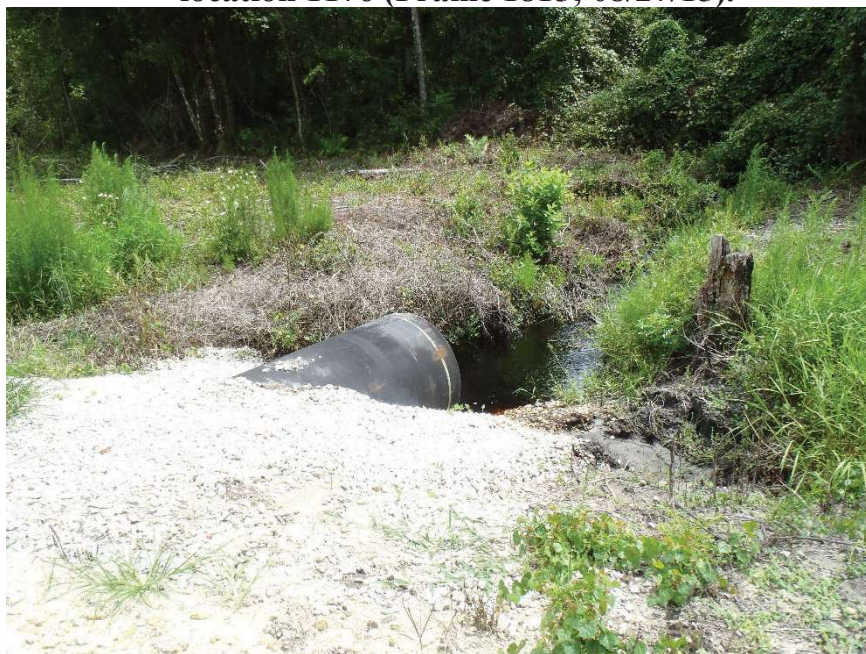
Photo 163. View of Physical Feature: Culvert located on south side of power line easement at GPS location 1176 (Frame 1816; 08/27/15).
