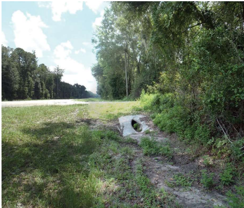
Photo 141. View of Physical Feature: Culvert as seen looking south from GPS location 1036 (Frames 1777-1778; 08/26/15).
