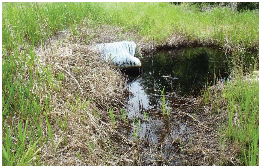
Photo 164. View of Physical Feature: Culvert located on north side of power line easement at GPS location 1177 (Frame 1817; 08/27/15).
