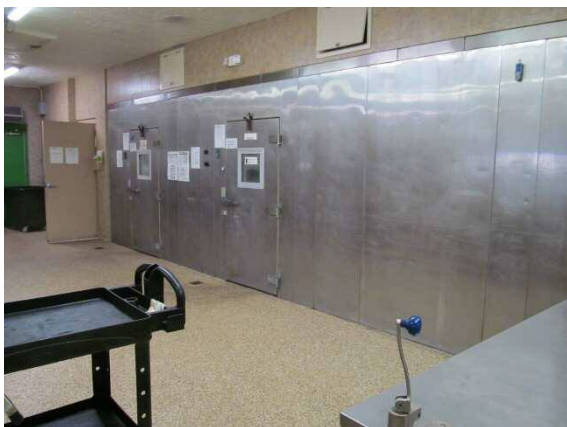
Building 11 kitchen area
