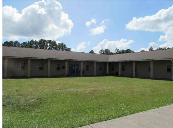
Building 7 Community Services Center (CSC)
