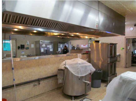
Building 11 kitchen area
