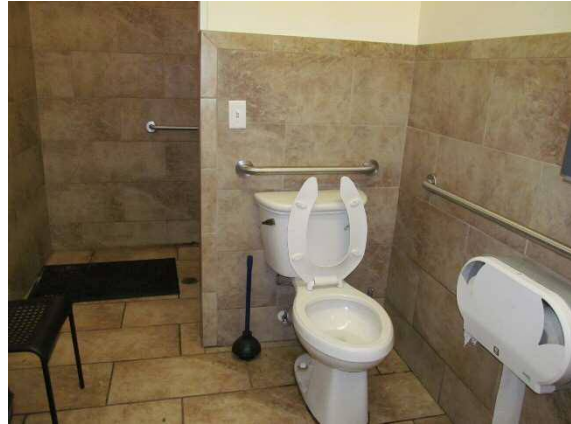
Building 12 typical restroom
