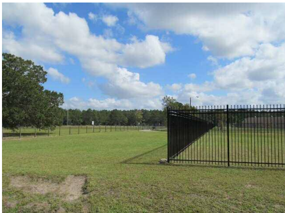
Typical site view perimeter fencing
