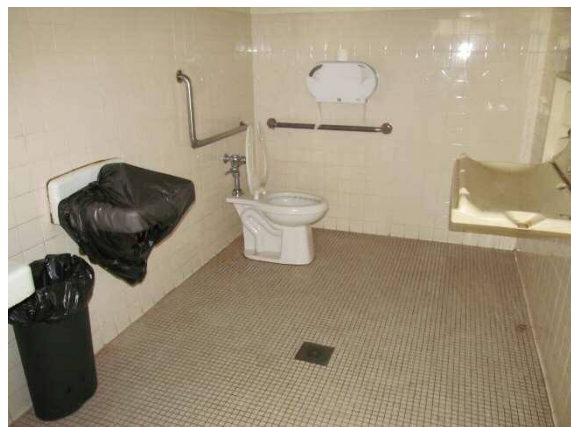
Building 13 typical restroom
