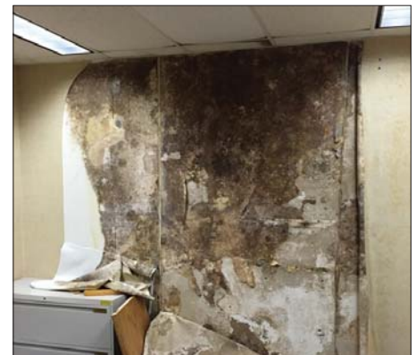
Mold Beneath Wall Coverings
