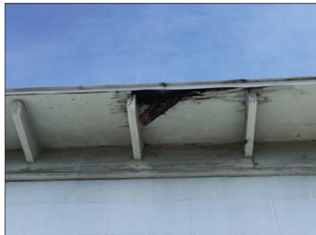
Rotten Wood At Roof Eave
