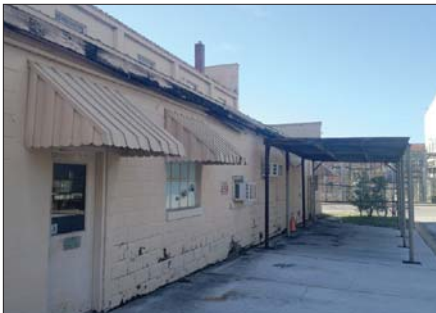
Deteriorating Exterior Paint On CMU
