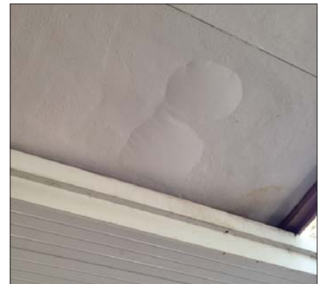
Damage Indicating Possible Roof Leak
