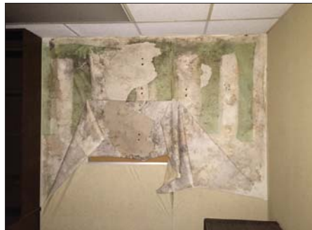
Mold Growth On Interior Wall
