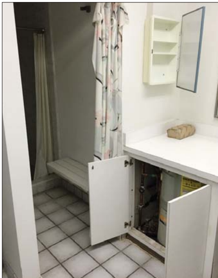
Toilet Room With Under-Counter Water Heater
