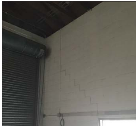
Wall Cracking
