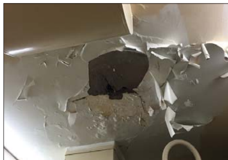
Water Damage Due To Roof Leak
