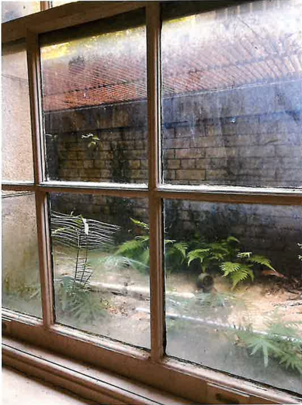
The pits outside the basement windows flood and have created water intrusion problems at the windows.
