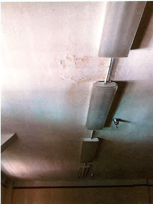
One of the areas with water intrusion evidence.
